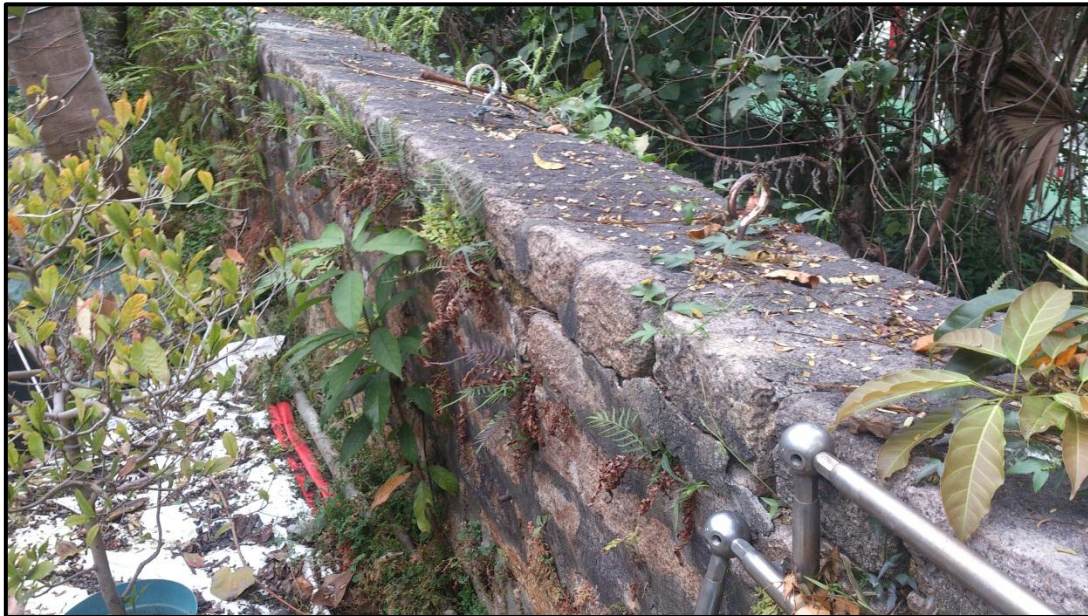
Figure 3: Existing Old Stone Wall with Mortar Joints
