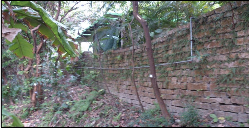
Figure 2: Existing Old Stone Wall without Mortar Joints
