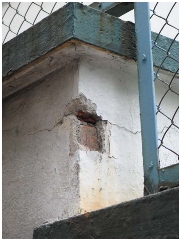
Exposed red bricks on the intermediate post of Aberdeen Street boundary wall
