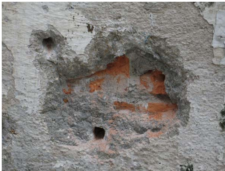
Exposed red bricks on the intermediate bay of Staunton Street boundary wall
