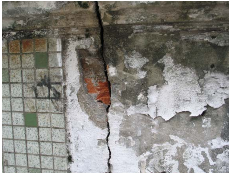
Exposed red bricks on Staunton Street boundary wall above the underground public latrine
