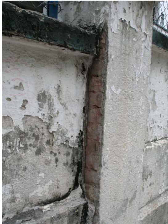
Exposed red bricks on the intermediate post of Staunton Street boundary wall
