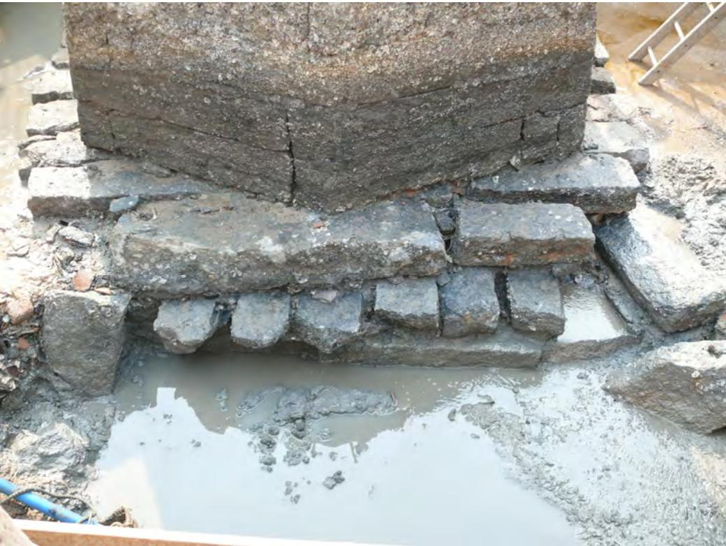
**Figure 47** Three Layers of Footing Stones of SP6 (View From East)
