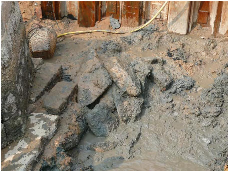
**Figure 53 Cobber Layer of SP6**
