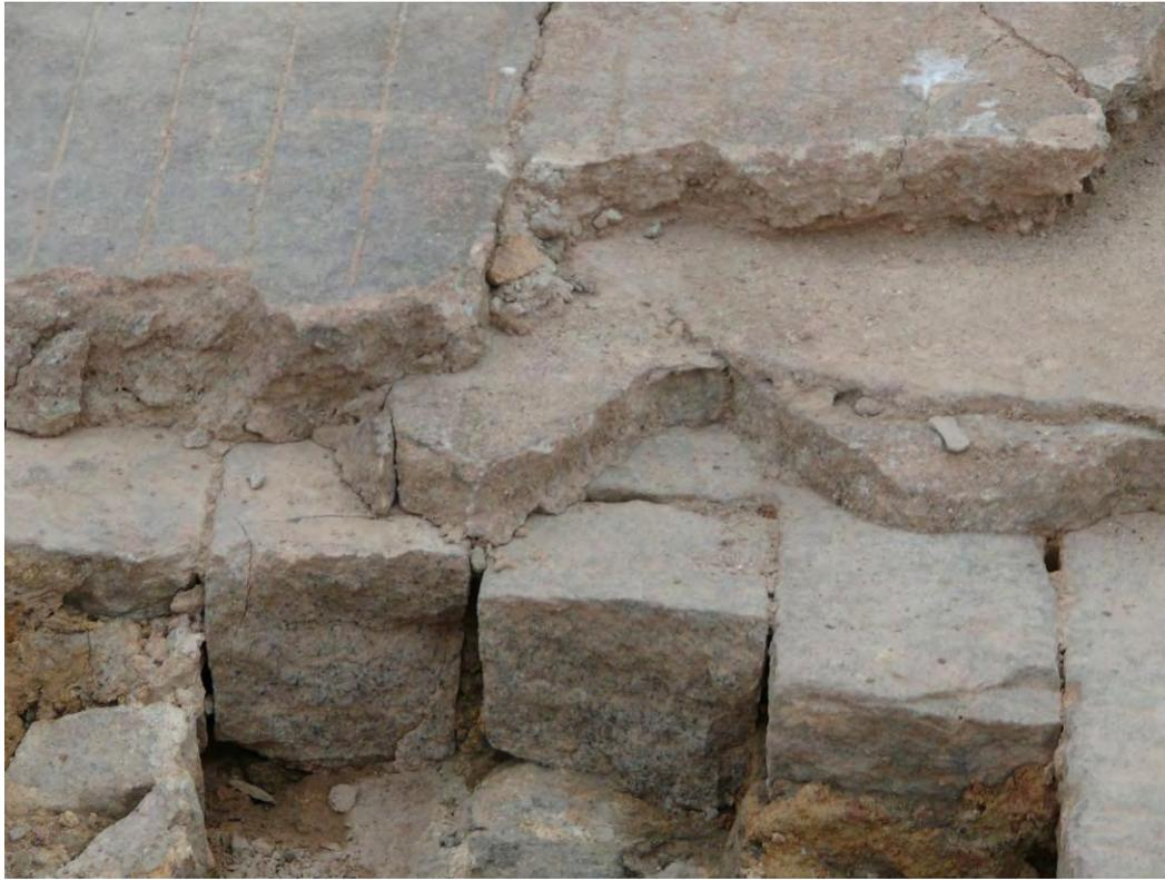
**Figure C7** Three Layers of Seaward End of Longjin Bridge
