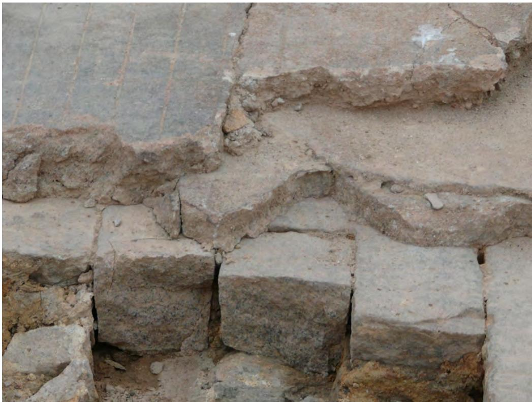
**Figure 30** Three Layers of Seaward End of Longjin Bridge
