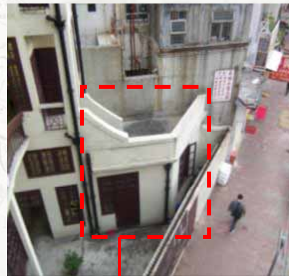
Servant Annex to be demolished for new fire escape stair so that openness of rear courtyard can be maintained
