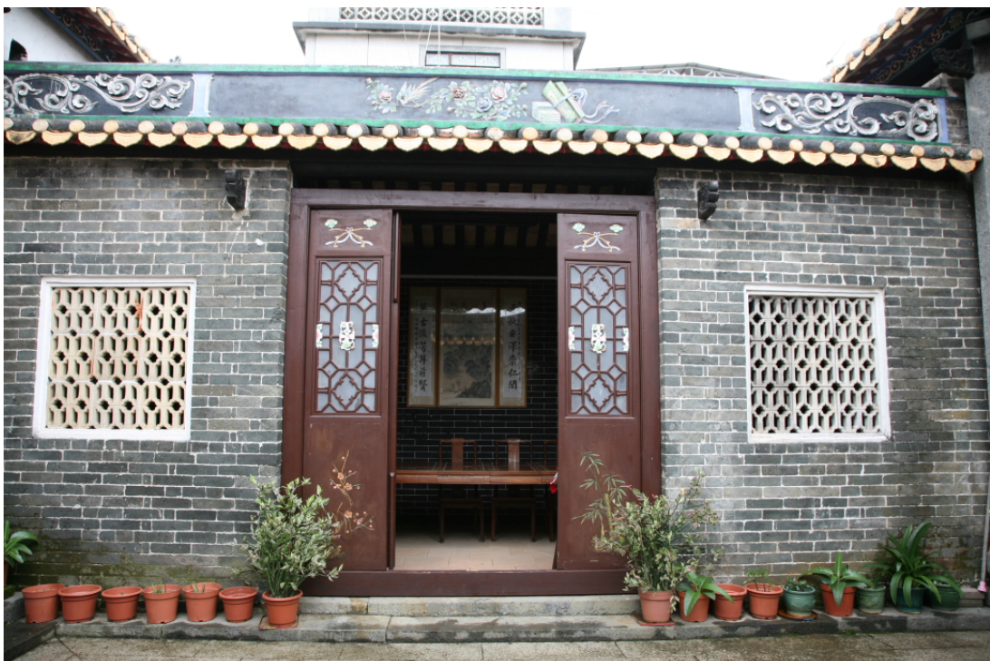
The wooden latticed doors and ceramic window grilles of the side chamber
