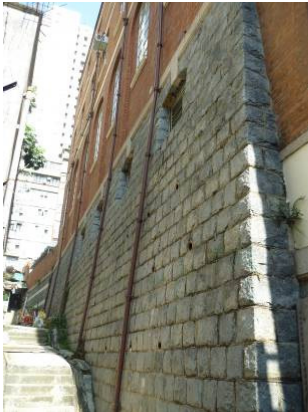
承托北翼的舊花崗石擋土牆
