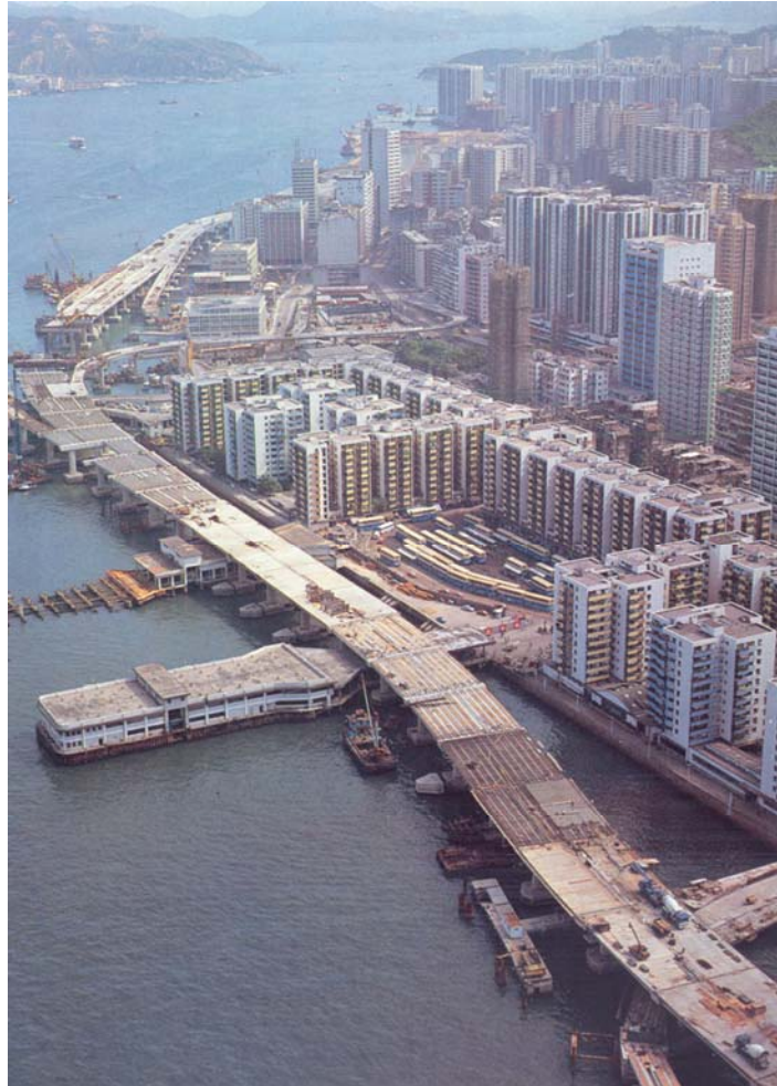
Fig. 48. Work in progress on the deck of the elevated carriageway in North Point. A large scale bus terminal was constructed adjacent to the North Point Ferry Pier. (from Highways Office, Engineering Development Department, Hong Kong Island Eastern Corridor: Causeway Bay to Taikoo Shing Section , Hong Kong, the Government Printer, 1984, p. 6)
