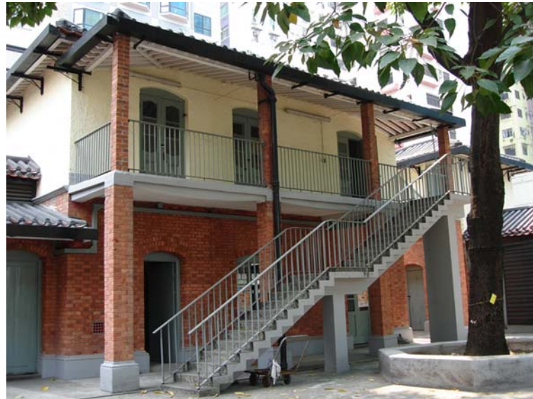
Fig. 156. Brick columns at the verandah of Annex A.
