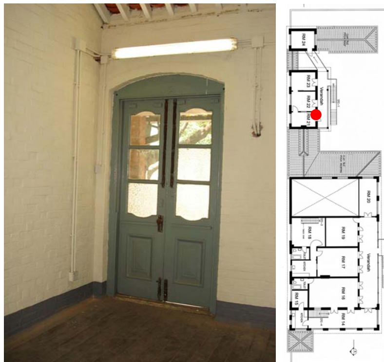
Fig. 396. Glazed timber French door at RM 21 of Annex A.
