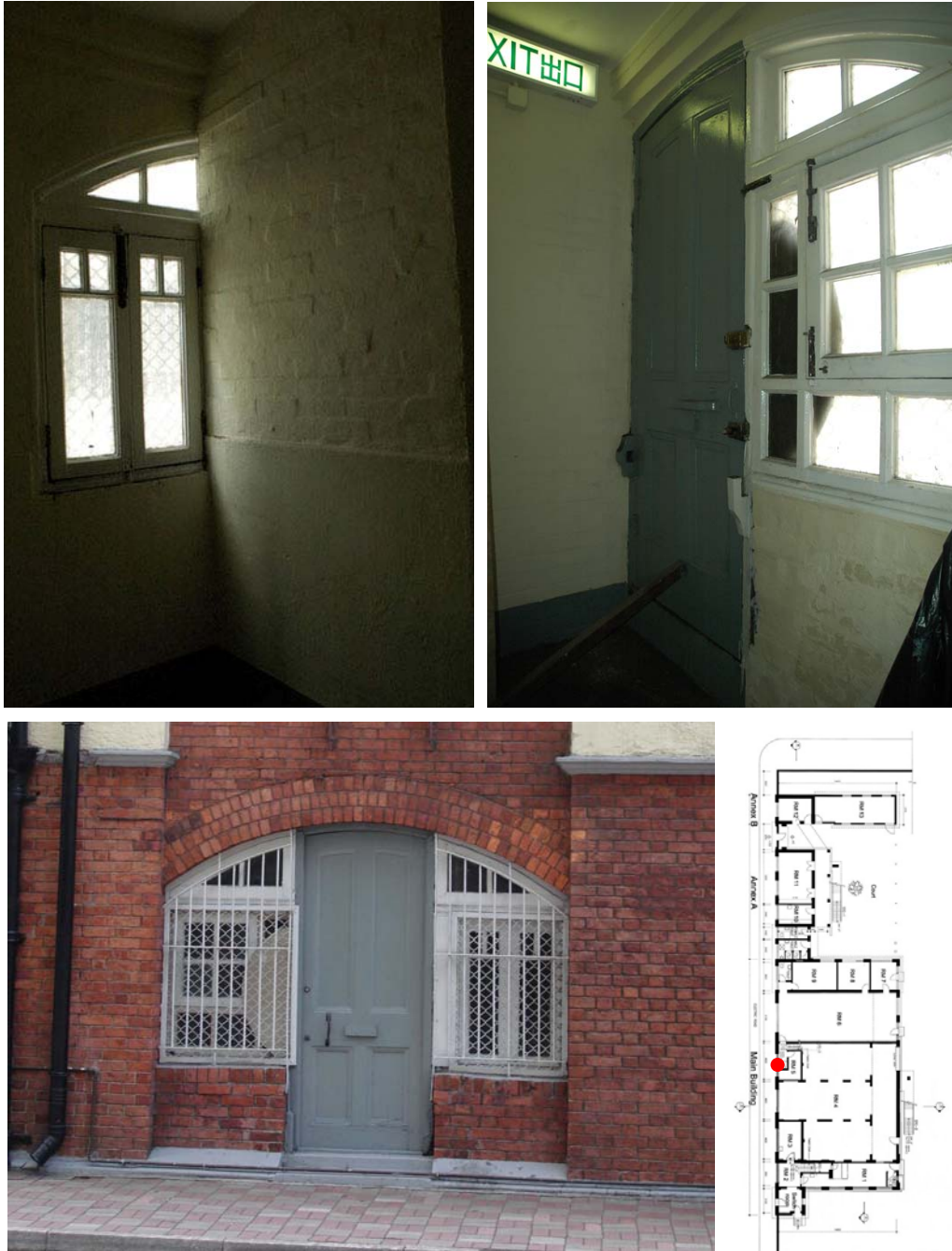
Fig. 273. The original segmental-headed window with door at the middle at RM 5 from the interior (above) and from the exterior (below) of the main building.
