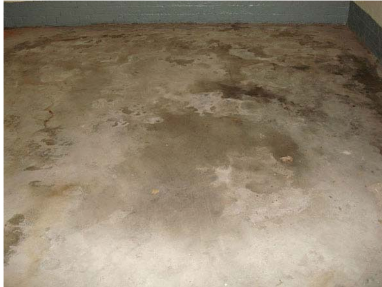
Fig. 294. Cement sand flooring of RM 7.
