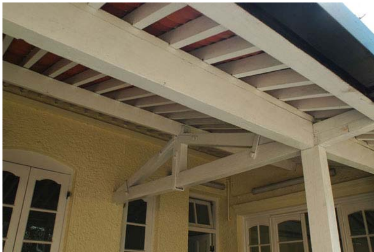
Fig. 321. Exposed roof trusses of the verandah at the main building.
