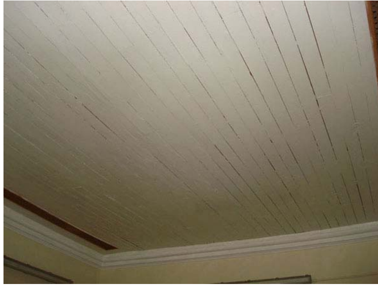
Fig. 358. Timber planks false ceiling at RM 19.
