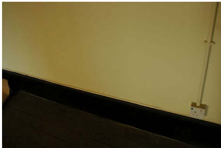
Fig. 341. Timber planks flooring with skirting of RM 17 at the main building.
