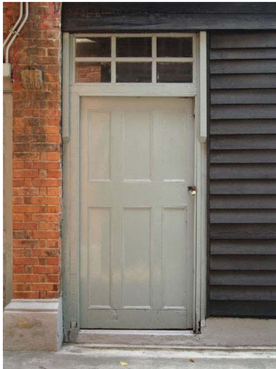
Fig. 431. Timber panelled door at the entrance of RM 13 of Annex B.
