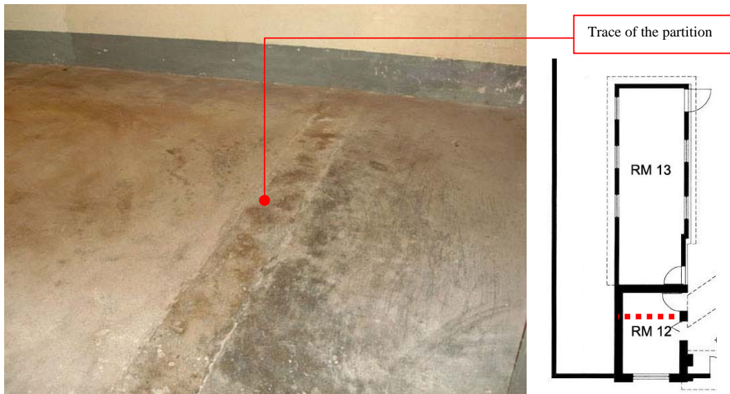
Fig. 421. Cement sand flooring of RM 12 at Annex B.
