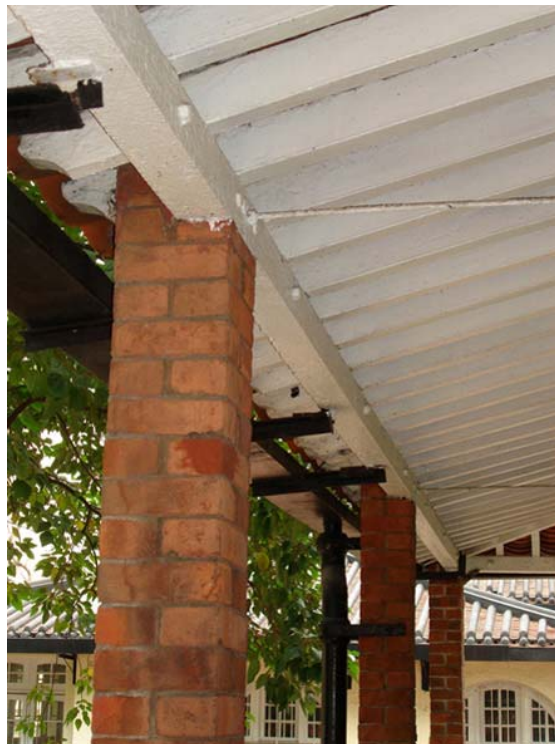
Fig. 373. Roof structure supported on brick columns at the verandah of Annex A.
