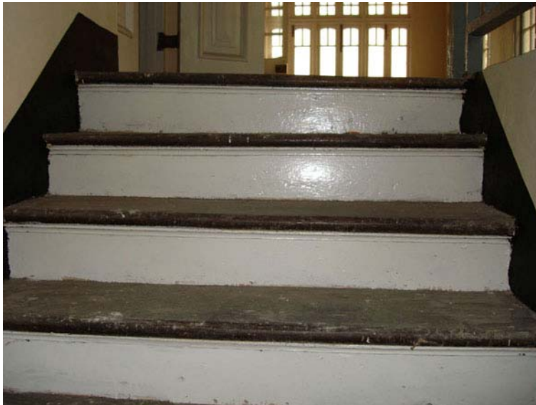
Fig. 242. Close up of the treads and risers of the timber staircase (STC – 4) at the main building.
