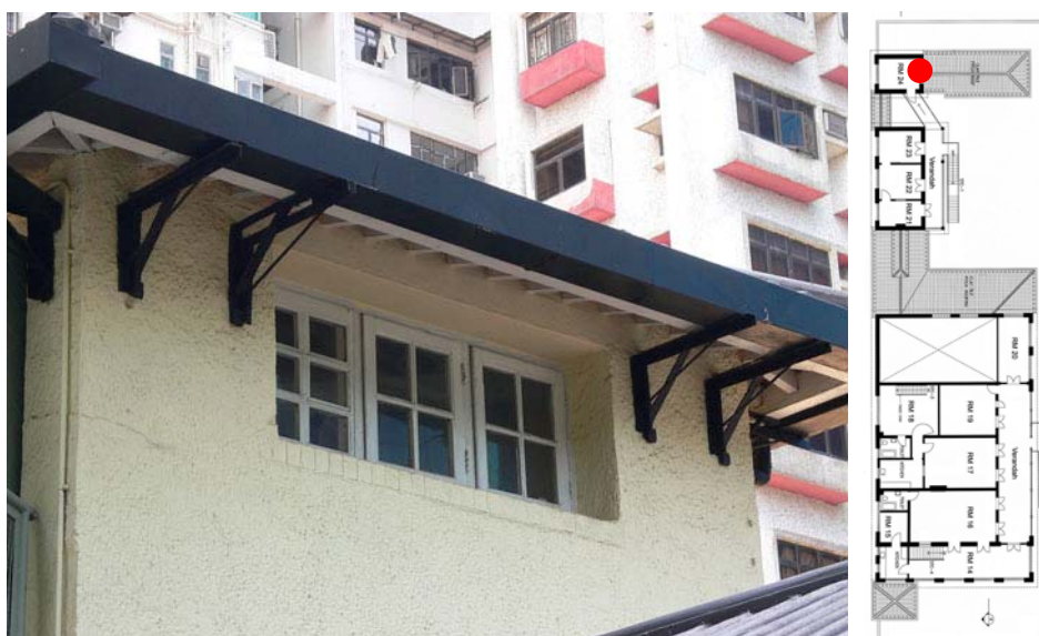
Fig. 440. Timber-framed windows on the rear façade at RM 24 of Annex B.
