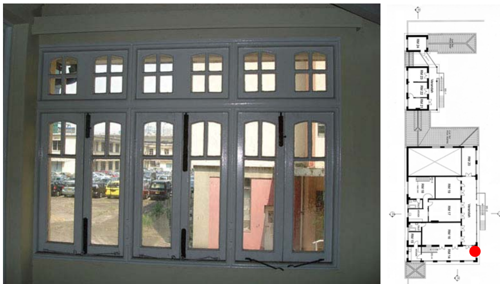
Fig. 313. Glazed timber windows at RM 14 of the main building.
