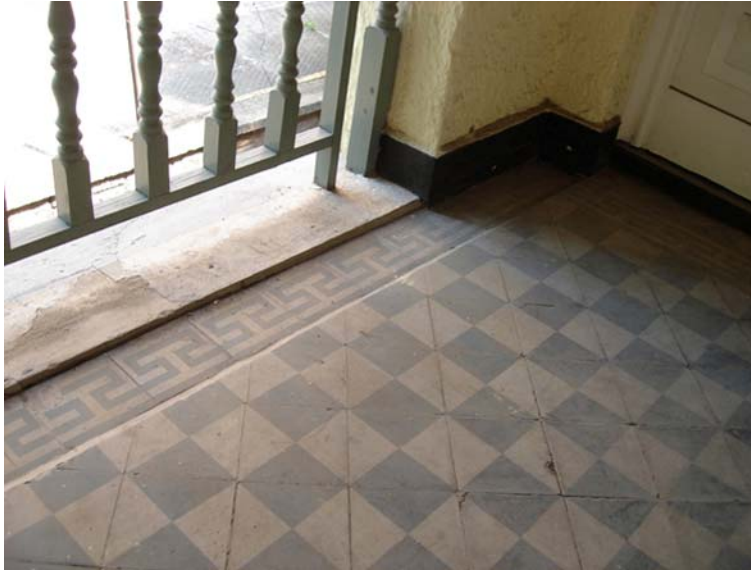
Fig. 322. Encaustic tiles with border and floor drain at the verandah of the main building.
