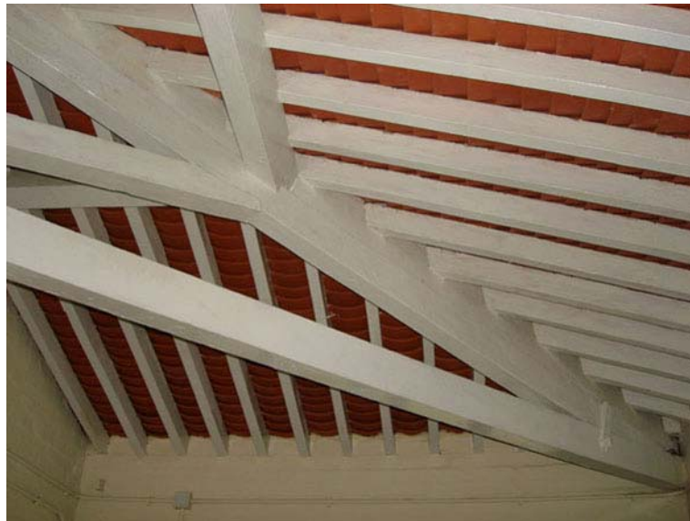
Fig. 291. Exposed roof structure at RM 7.
