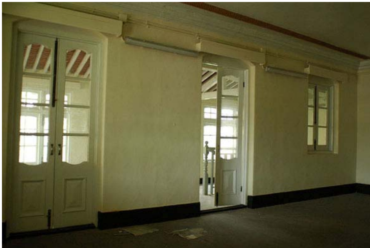
Fig. 332. Glazed timber French doors and casement windows at RM 16 of the main building.
