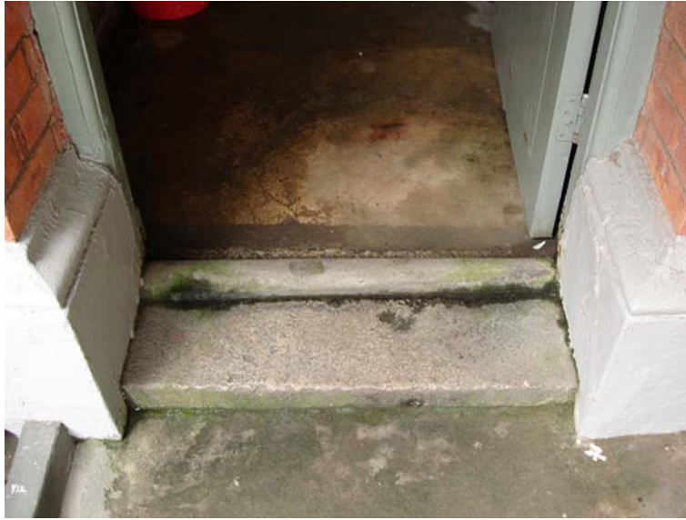
Fig. 417. Granite threshold at the doorway of the female toilet at Annex A.
