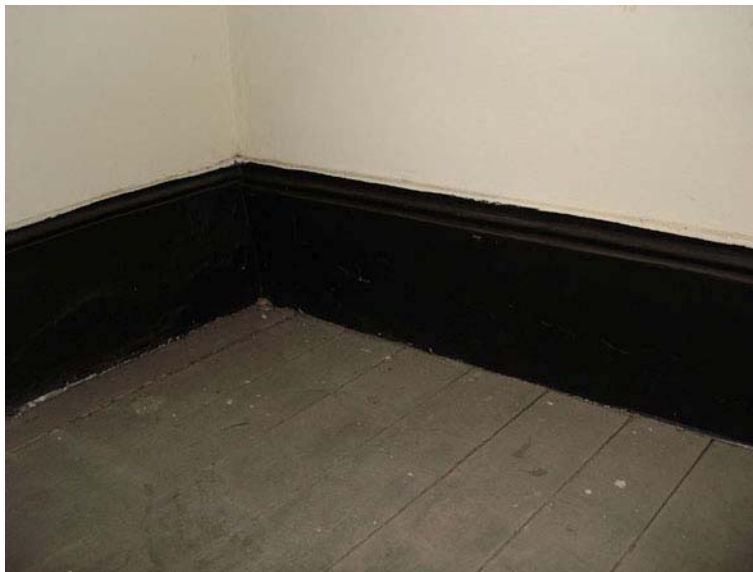
Fig. 328. Flooring with timber planks and skirting at RM 15 of the main building.
