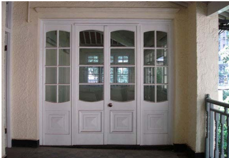
Fig. 365. Glazed timber French door to RM 20 at the main building.
