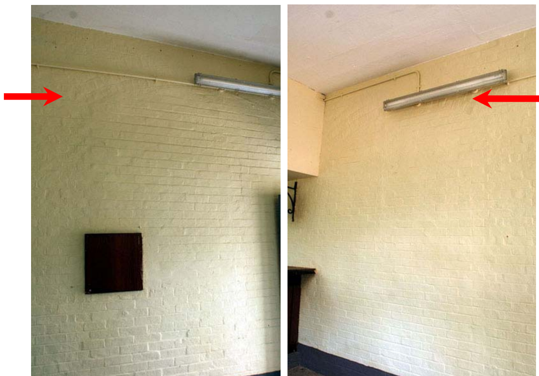
Fig. 253. Traces of the original archways on the wall at RM 1.
