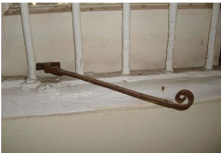
Fig. 367. Scrolled window stay of the window at RM 20 of the main building.
