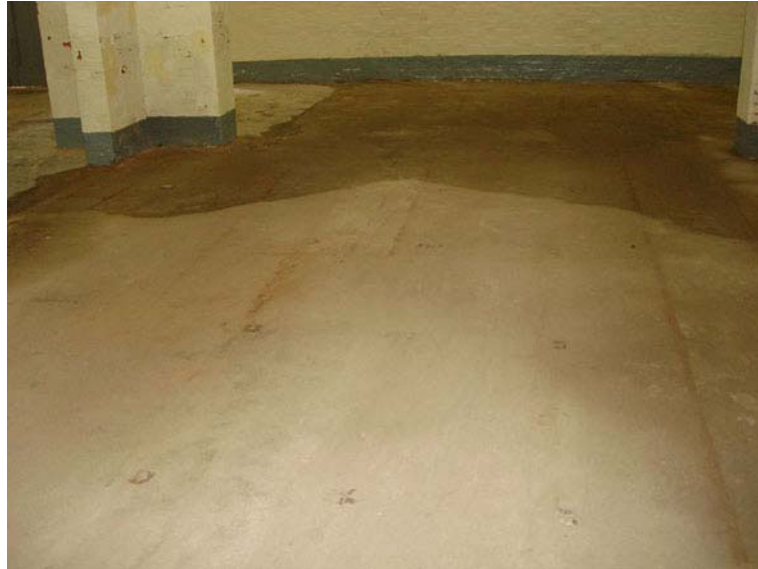
Fig. 263. Cement sand flooring of RM 4.
