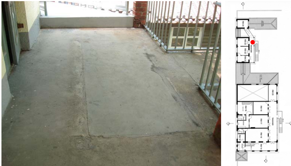
Fig. 100. Traces showing the location of the existing concrete staircase at the verandah on the first floor of Annex A.
