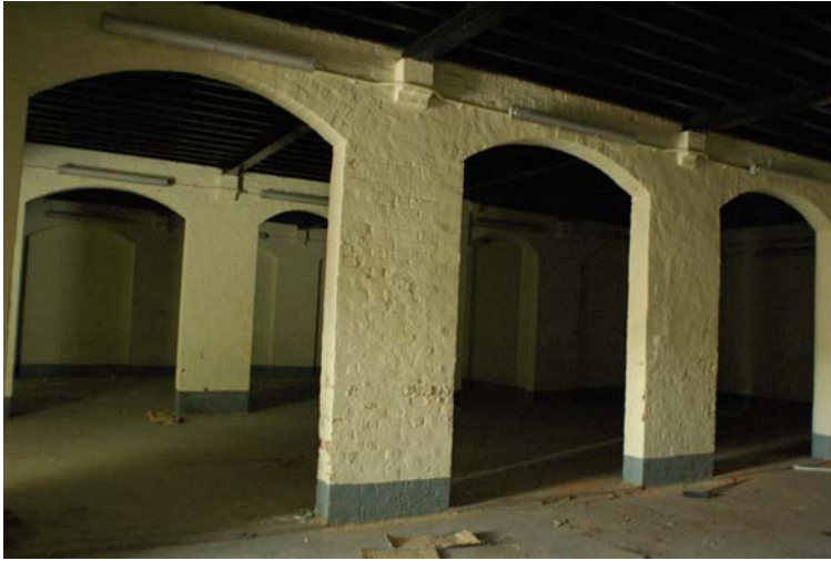
Fig. 165. Segmental archways at RM 4 on the ground floor.
