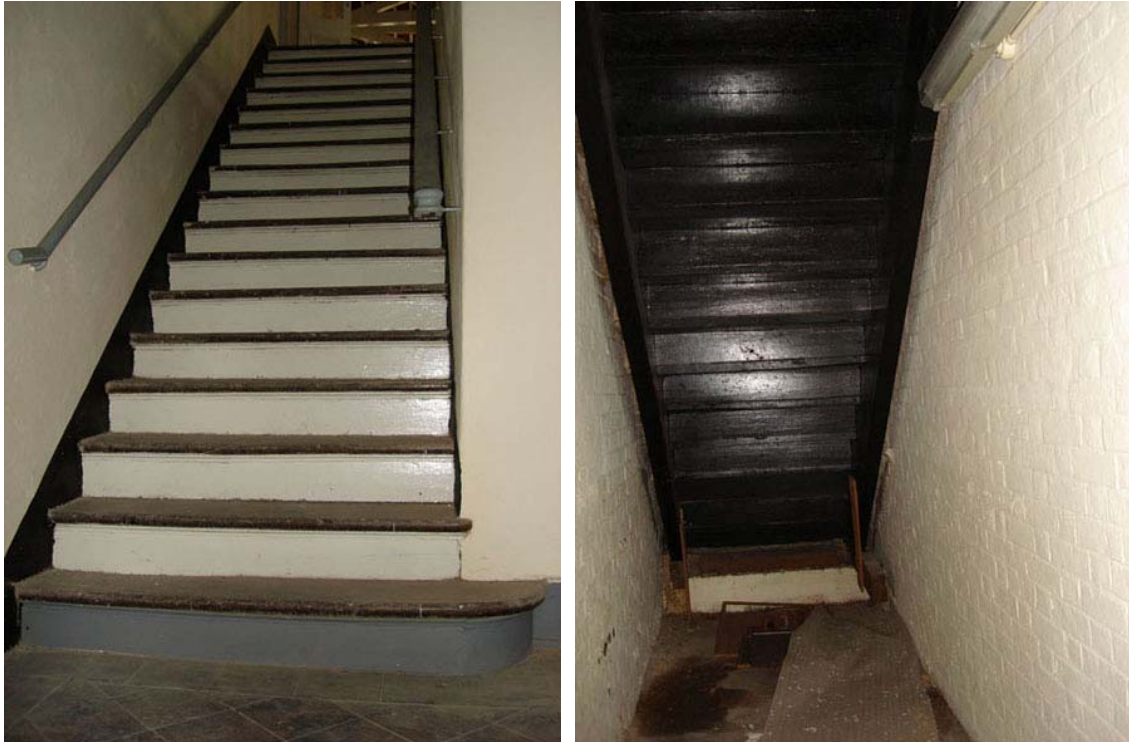
Fig. 239. Overview (left) and the underside (right) of the timber staircase (STC – 4) at the main building.
