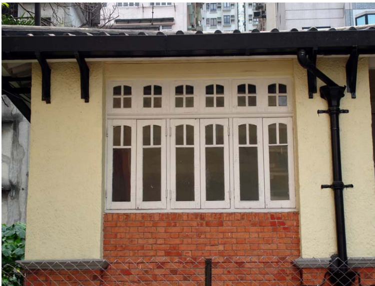
Fig. 166. Segmental-headed timber window glazings on the first floor at RM 14.
