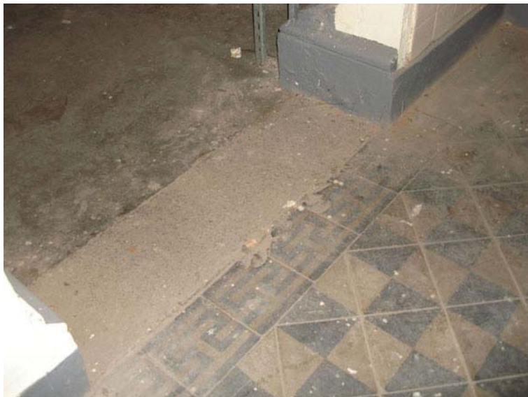
Fig. 232. Granite threshold between the former entrance porch and RM 2.
