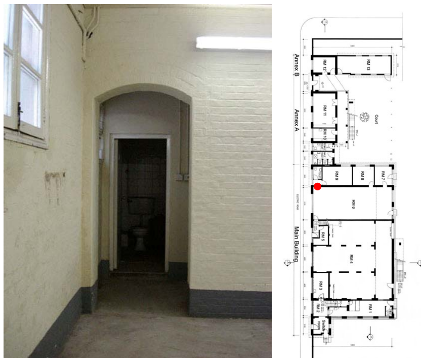
Fig. 301. Segmental-headed doorway to RM 9.
