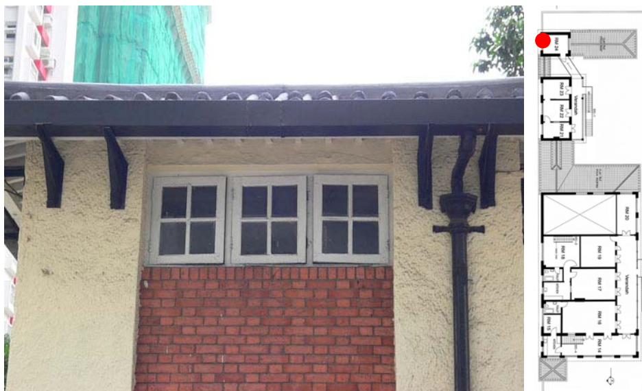
Fig. 439. Timber-framed windows on the front façade at RM 24 of Annex B.
