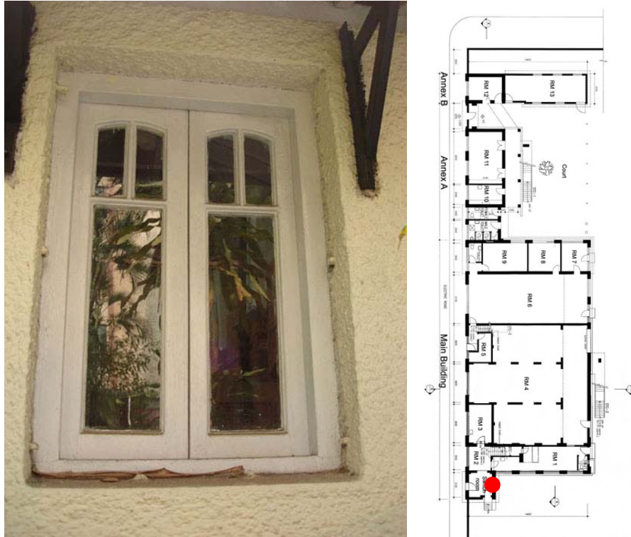
Fig. 228. Window with segmental-headed glazing at the former entrance porch.
