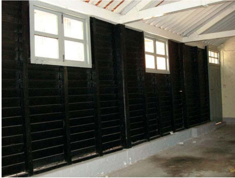
Fig. 427. Wall constructed with timber planks at RM 13 of Annex B.
