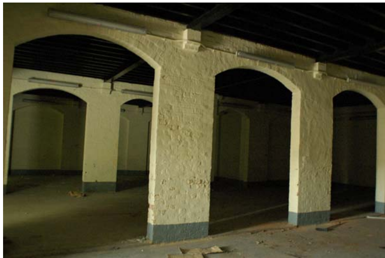
Fig. 259. Segmental archways at RM 4 of the main building.
