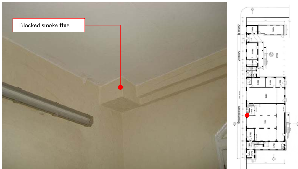
Fig. 276. Blocked smoke flue found in RM 5.
