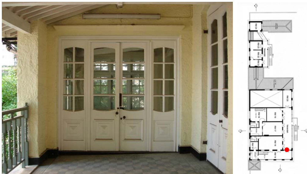
Fig. 315. Glazed timber French doors from RM 14 to the verandah at the main building.
