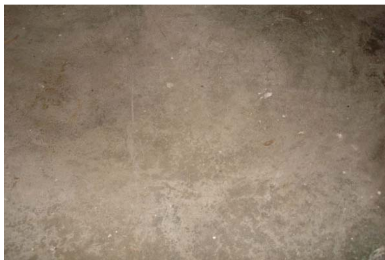
Fig. 233. Cement sand flooring of the former entrance porch.
