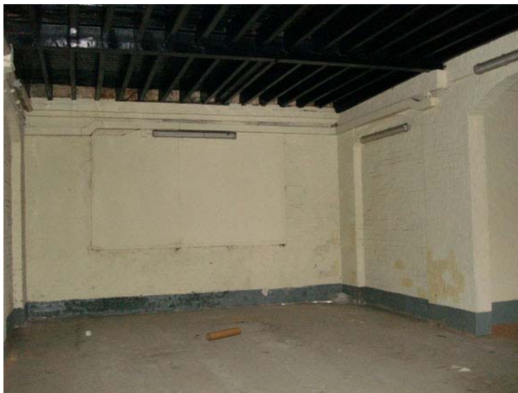
Fig. 264. Original segmental arched windows blocked at RM 4 of the main building.
