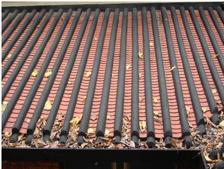
Fig. 158. Traditional double-layered roof of Chinese pan and roll tiles.
