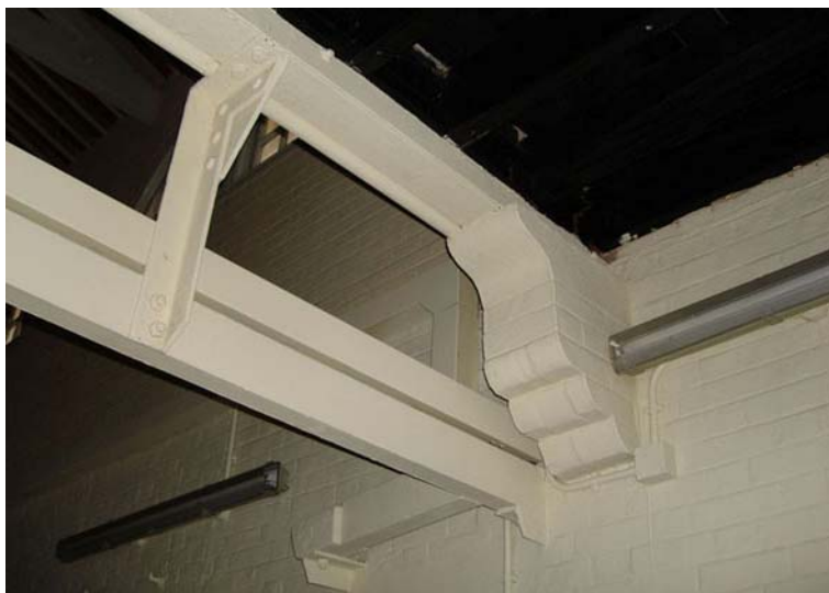
Fig. 286. Steel section supported on bracket at RM 6 of the main room.
