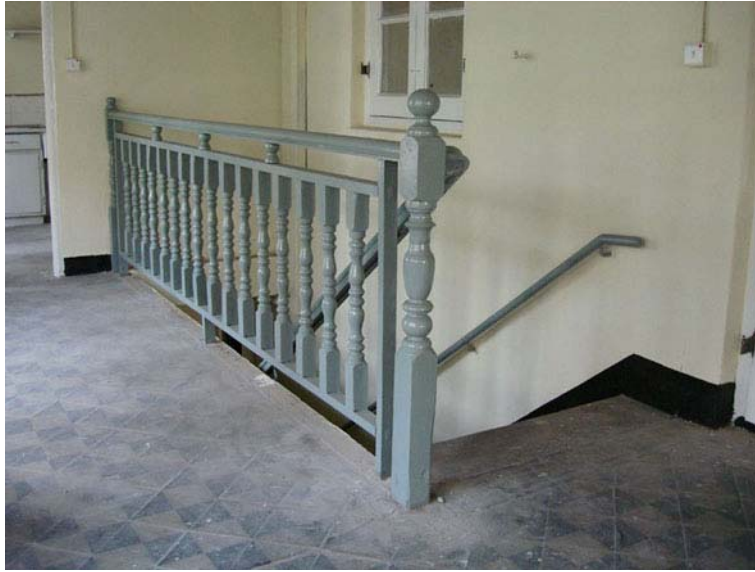
Fig. 241. Timber balustrade of the timber staircase (STC – 4) on the first floor of the main building.
