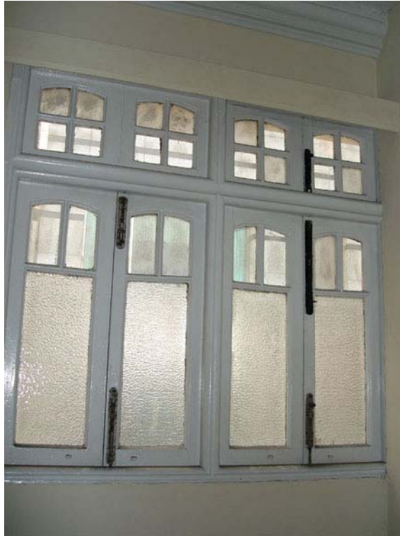
Fig. 327. Glazed timber casement windows at RM 15 of the main building.
