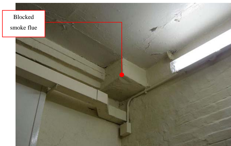
Fig. 249. The blocked smoke flue at RM 3.
