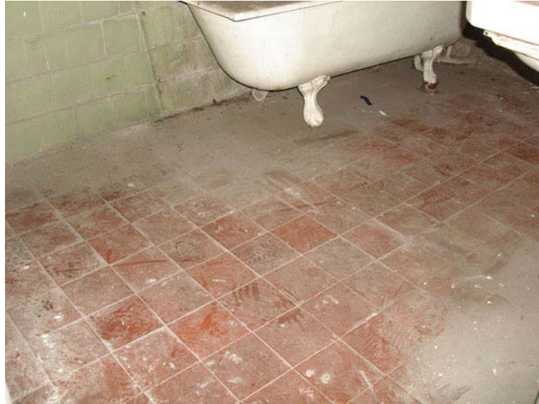
Fig. 354. Red quarry floor tiles at the bathroom of RM 18.
