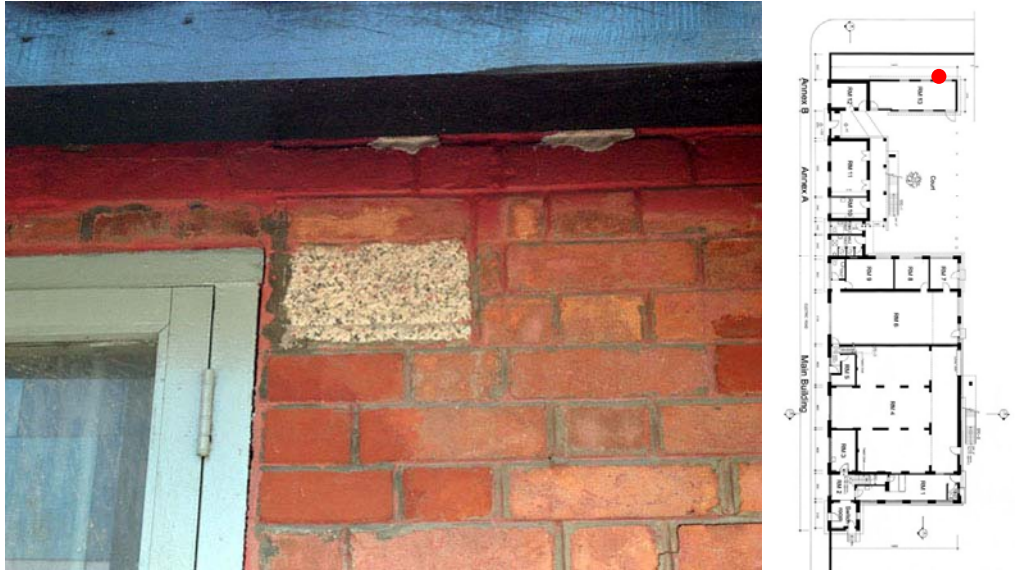
Fig. 429. Granite block for the support of timber roof truss at RM 13 of Annex B.
