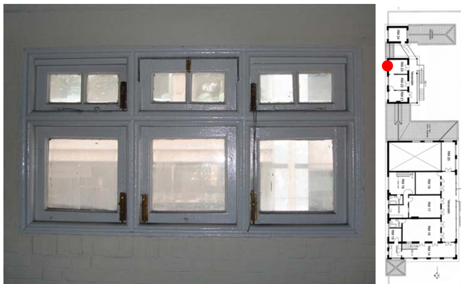
Fig. 408. Timber framed windows at RM 23 of Annex A.
