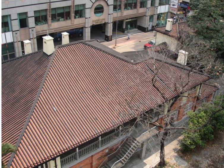
Fig. 157. Hipped roof of the main building.
