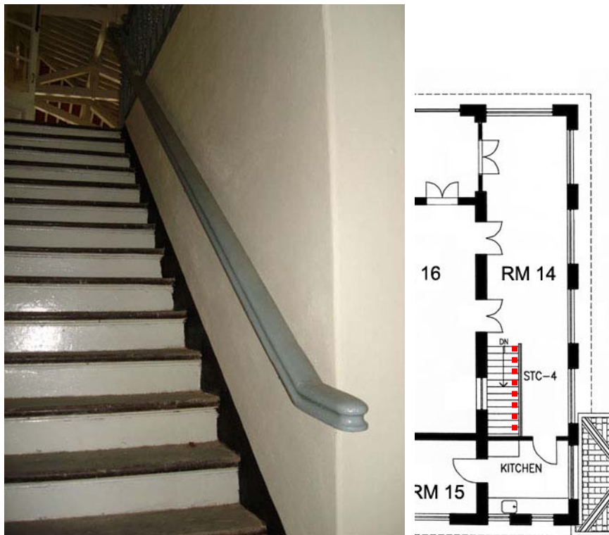
Fig. 240. The handrail of the timber staircase (STC – 4) at the main building.
