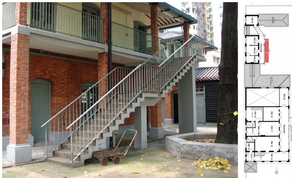
Fig. 379. Concrete staircase (STC – 1) at the rear of Annex A.
