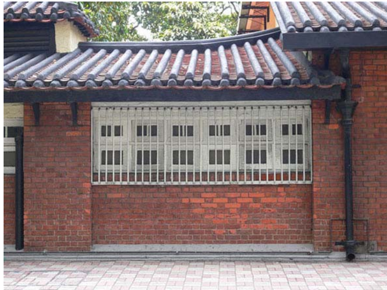
Fig. 307. Timber-framed windows of the toilet to RM 6 on the front façade.
