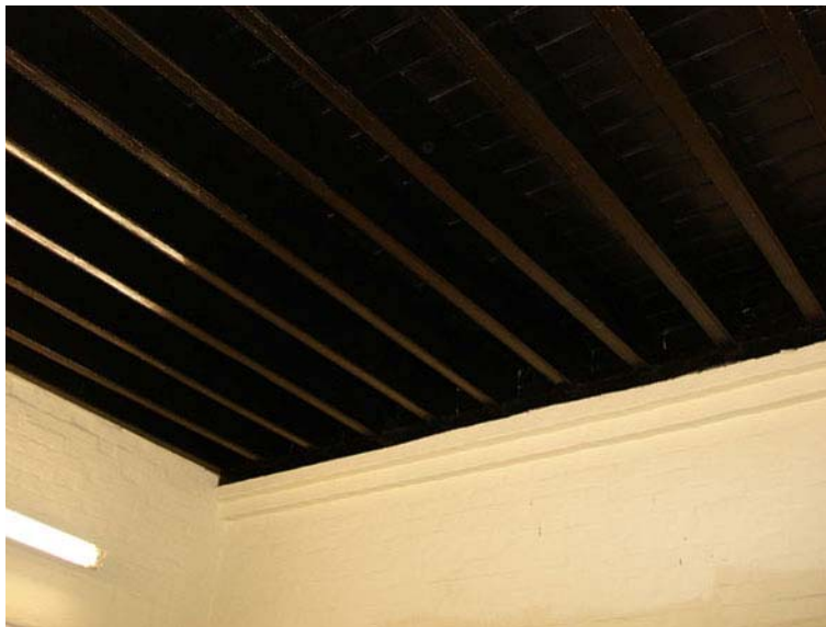
Fig. 420. Exposed timber structure of the ceiling at RM 12 of Annex B.
