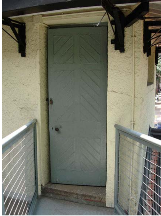
Fig. 437. Framed, ledged and braced battened door at the entrance of RM 24 at Annex B.
