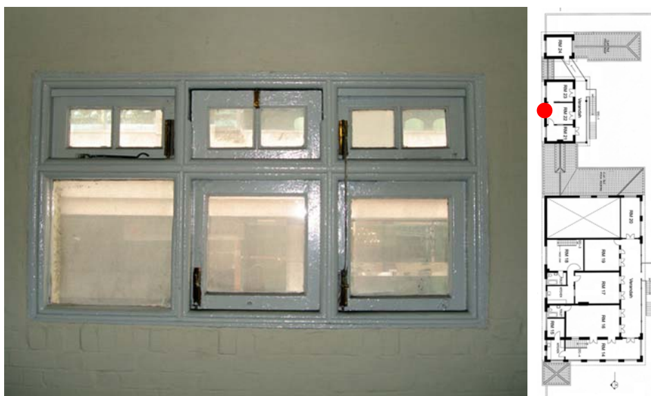
Fig. 402. Timber-framed windows at RM 22 of Annex A.
