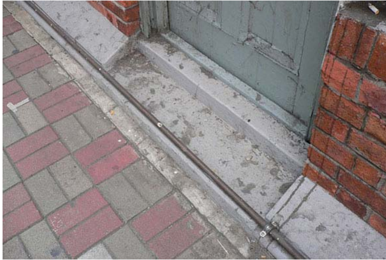
Fig. 185. Hidden plinth at the front façade of the main building.
