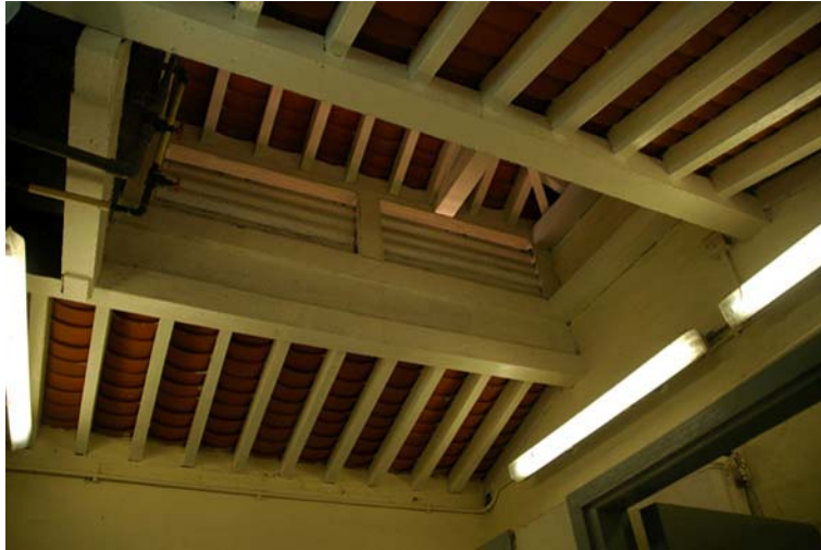
Fig. 413. The exposed structure of the vent at the male toilet of Annex A.
