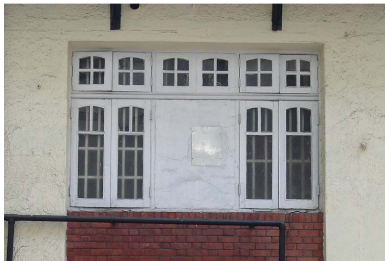
Fig. 347. Casement windows viewed from the front façade.
