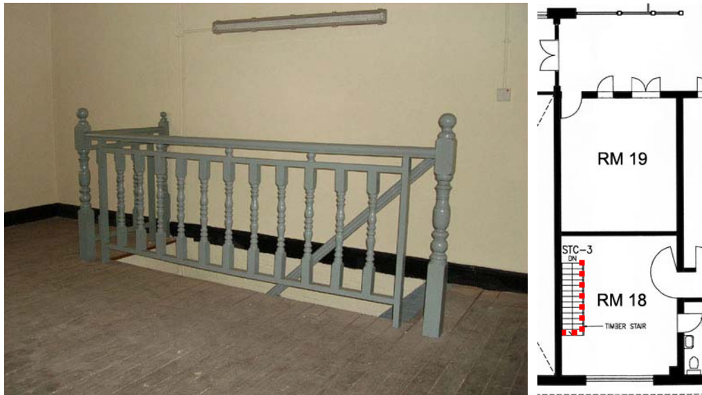
Fig. 280. Timber balustrade of the timber staircase (STC – 3) at the main building.
