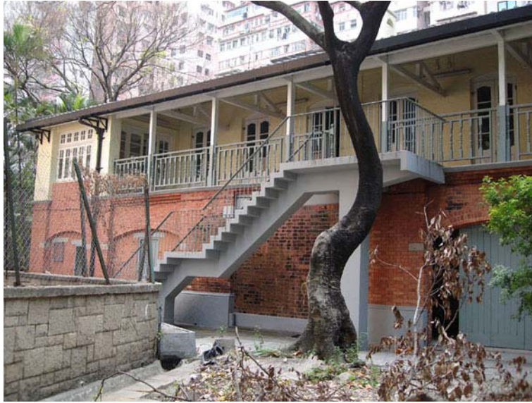
Fig. 269. The concrete staircase (STC – 2) at the main building.
