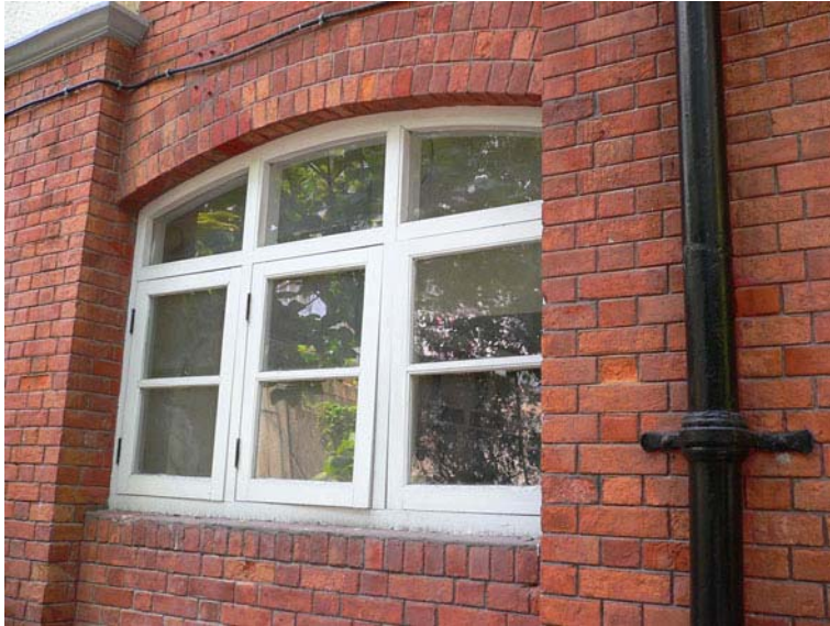
Fig. 208. Later added timber-framed window at RM 1 on the ground floor.
