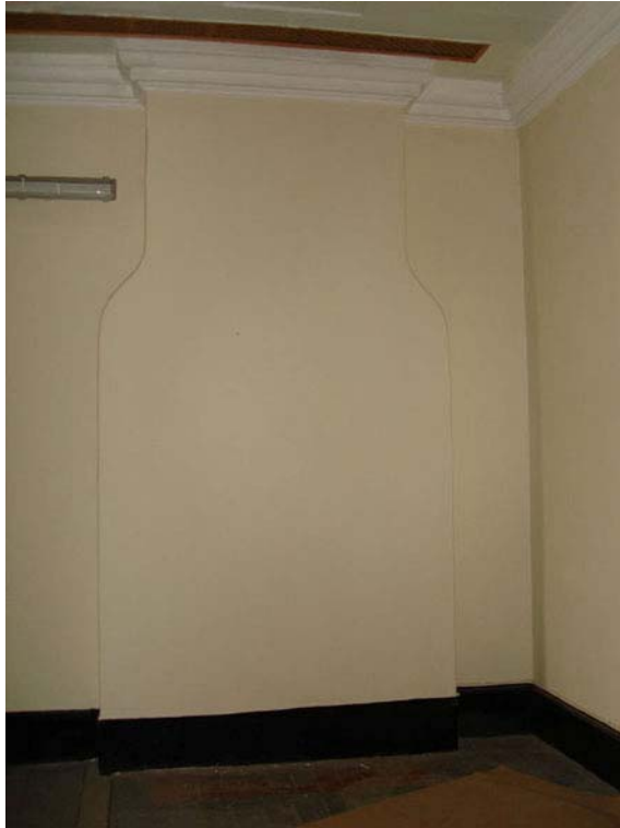
Fig. 343. Chimney breast of RM 17 at the main building.
