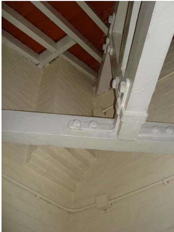
Fig. 293. Close up of the original smoke flue at RM 7 of the main building.
