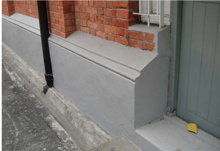
Fig. 198. Tall and thick plinth at the rear façade of the main block.
