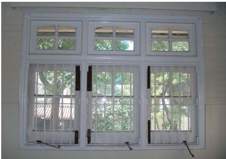
Fig. 366. Glazed timber windows at RM 20 of the main building.
