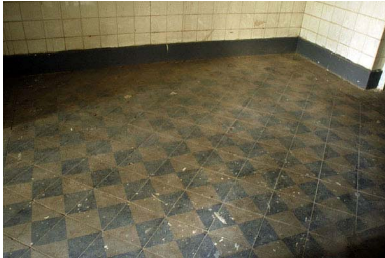
Fig. 237. Encaustic flooring tiles of RM 2.
