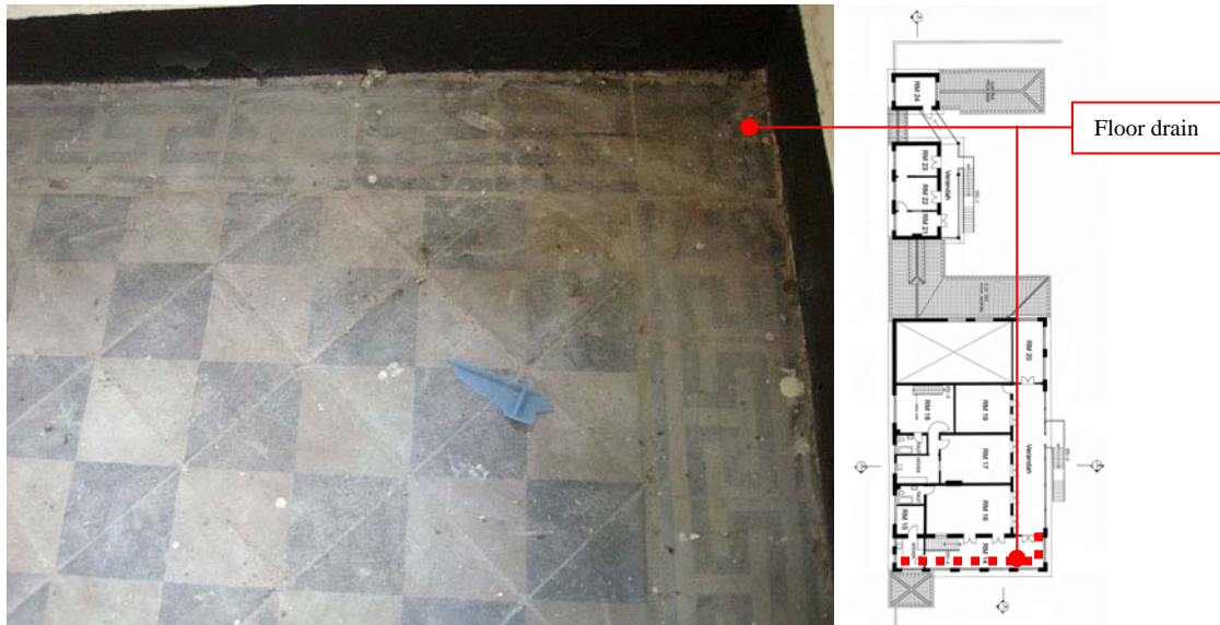
Fig. 312. Encaustic flooring tiles with border of RM 14 at the main building.
