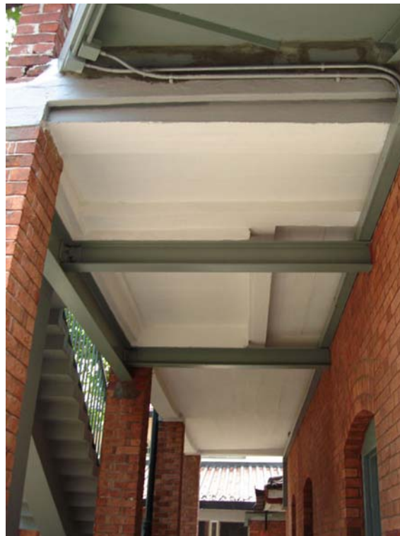
Fig. 101. Traces of the stair well from the ceiling of the arcade below.
