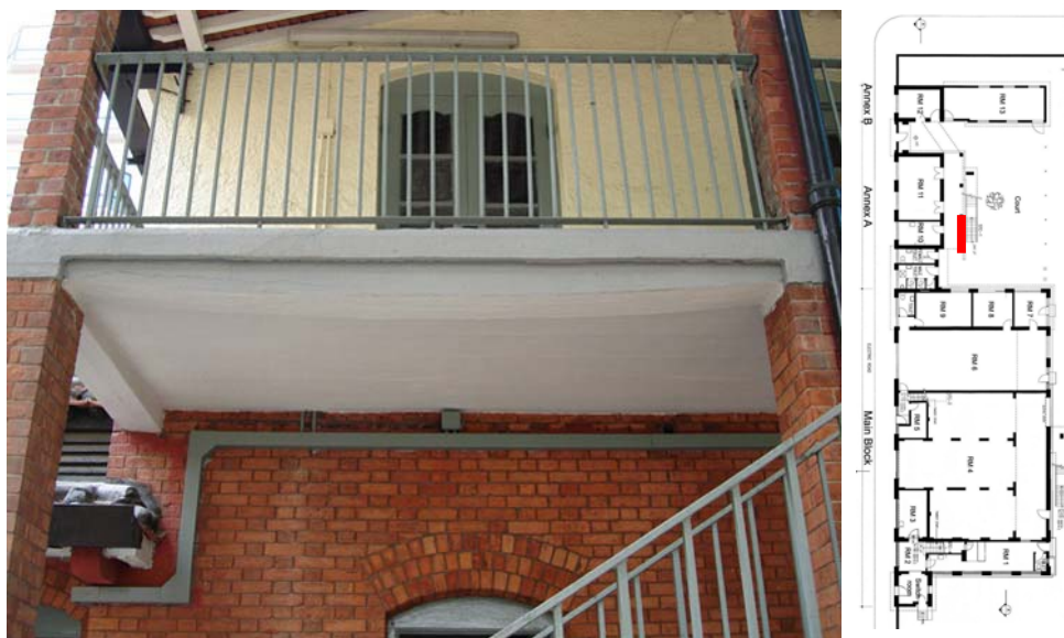
Fig. 371. Curved beam at the colonnaded arcade at Annex A.
