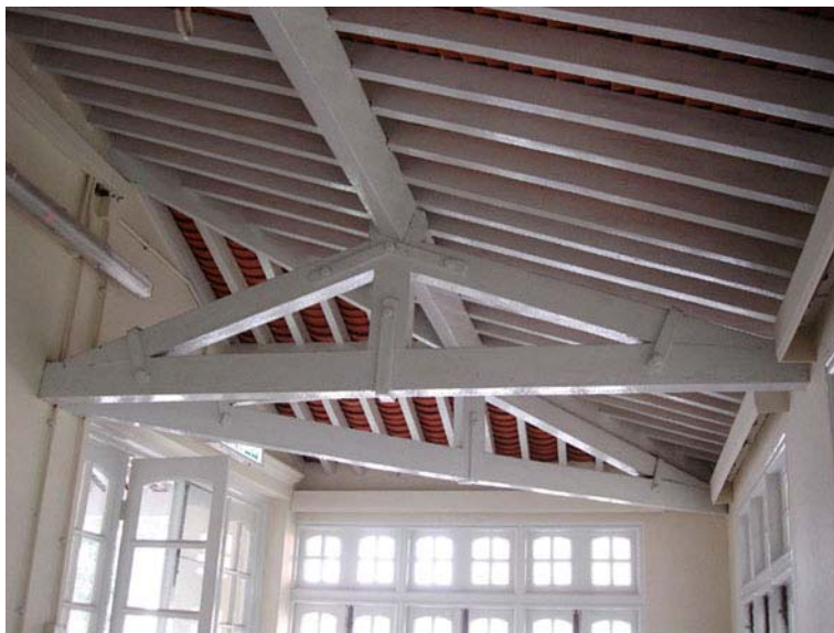
Fig. 311. Exposed roof structure of RM 14 at the main building.
