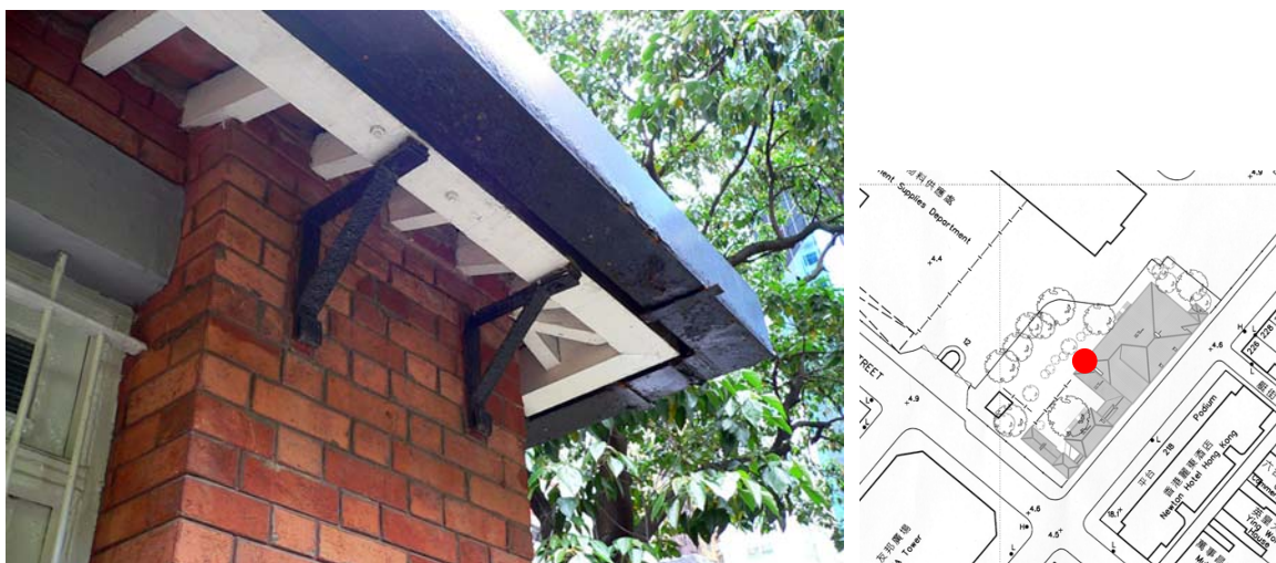
Fig. 154. Iron brackets under the eaves of the main building.
