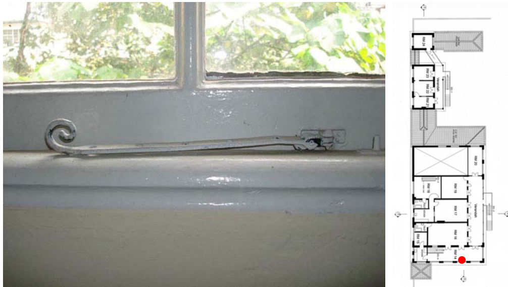
Fig. 314. Scrolled iron window stay at RM 14 of the main building.
