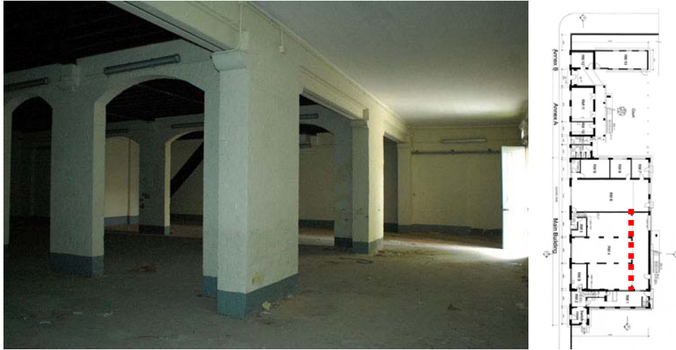
Fig. 261. Piers with brackets holding steel beams at RM 4 at the main building.
