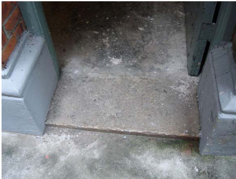
Fig. 423. Granite threshold at the entrances of RM 12 of Annex B.
