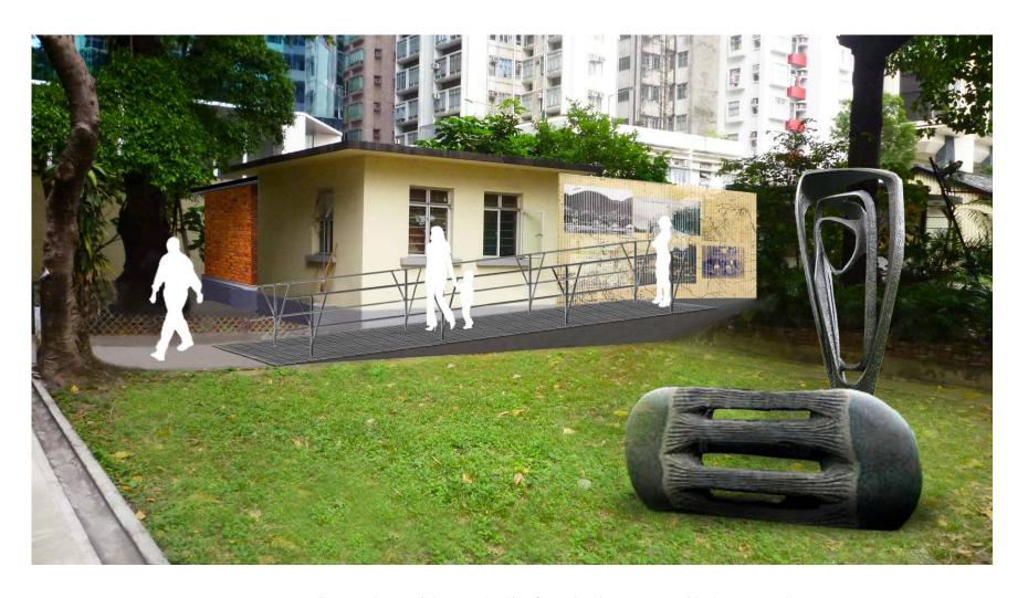
Proposed accessible ramp leading from the site entrance with the proposed combined F.S. and sprinkler tank beside the existing guard house, which would be screened off by decorated panels.
