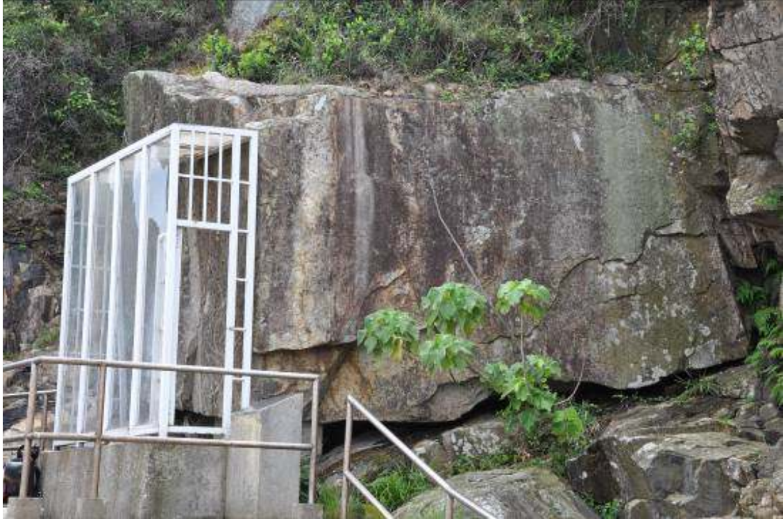
Figure 62. View of the block from the lateral side. Note the large overhang underneath it.
