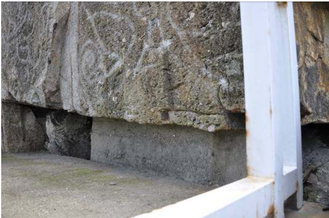
Figure 63. Detail of the cement pillars placed under the overhang
