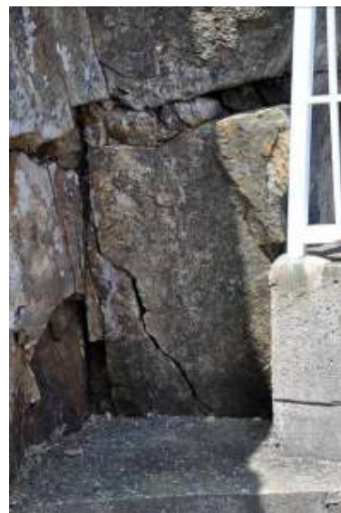
Figure 64. Detail of a crack at the base of the rock, on the left hand side.
