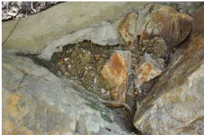
Figure 9. Detail of the lower part of the cement barrier. Note the space existing between the underlying soil and the cement. There are also visible cracks between the cement and the rock (upper right side)
