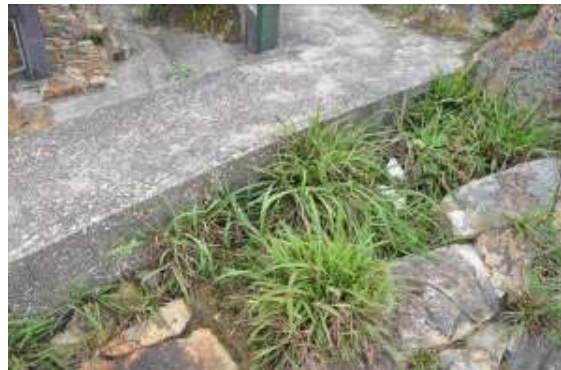
Figures 82 and 83. Details of the cement barrier above the engravings, and the vegetation growth on the channels removing water around the site.
