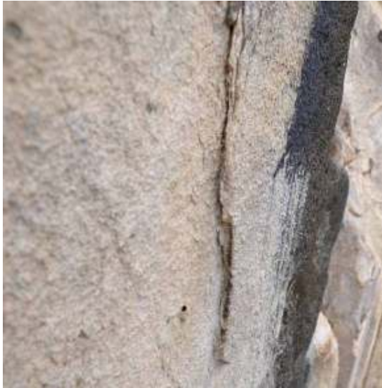
Figure 44. Detail of areas that should be monitored, to detect any possible risk of delamination
