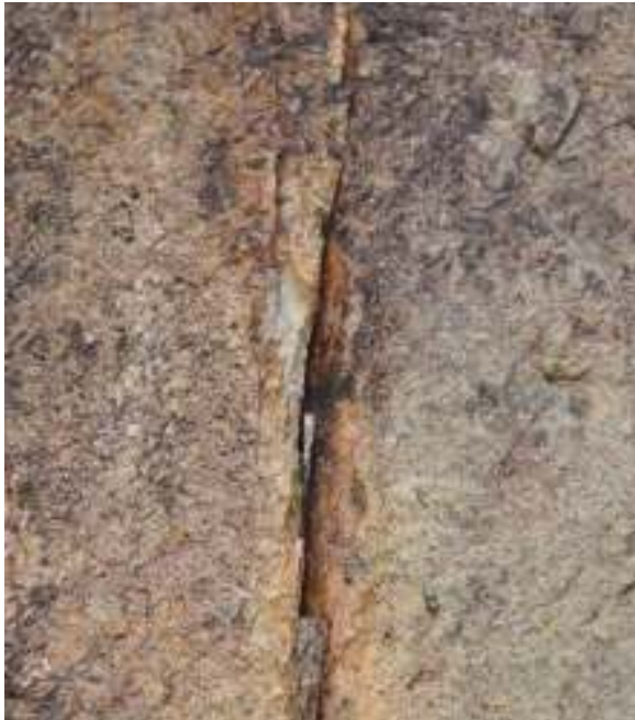
Figure 73. Detail of small scales on a vertical crack
