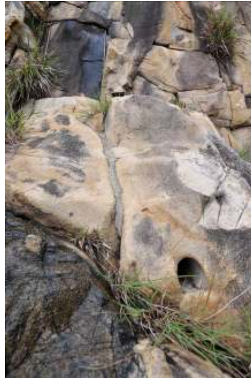
Figure 50. Detail of the drilled holes and the infills on the cracks
