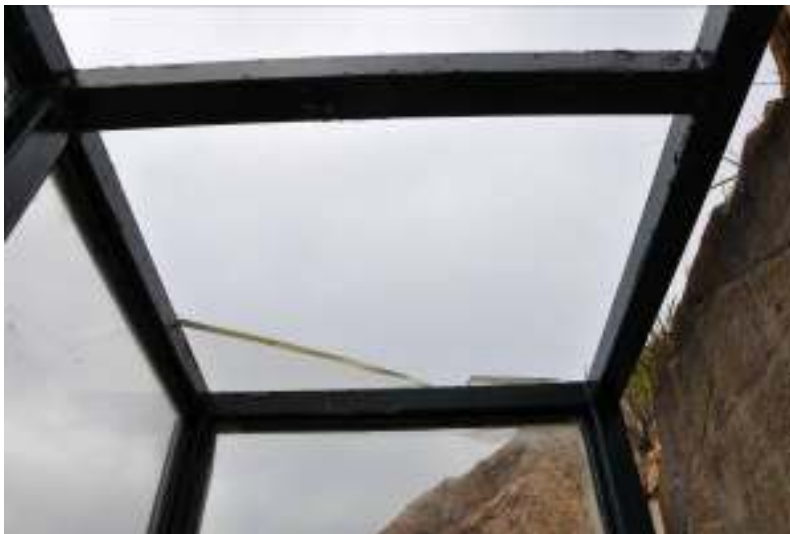
Figure 32. Detail of the upper broken glass
