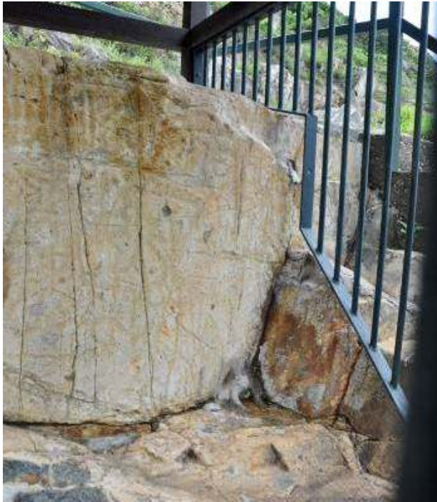
Figure 86. Detail of the right side of the site, with water seeping along a series of cracks
