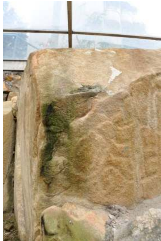
Figures 103 and 104. Detail of water seeping from the roof structure (left) and evidence of microorganisms growth under the roof railings
