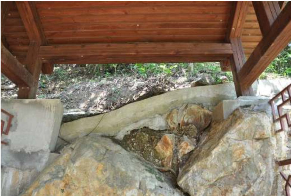
Figure 6. Cement channel on top of the shelter
