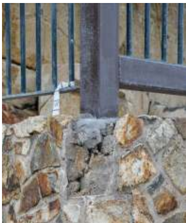
Figure 90. Detail of the corner of the viewing platform, with a missing stone.
