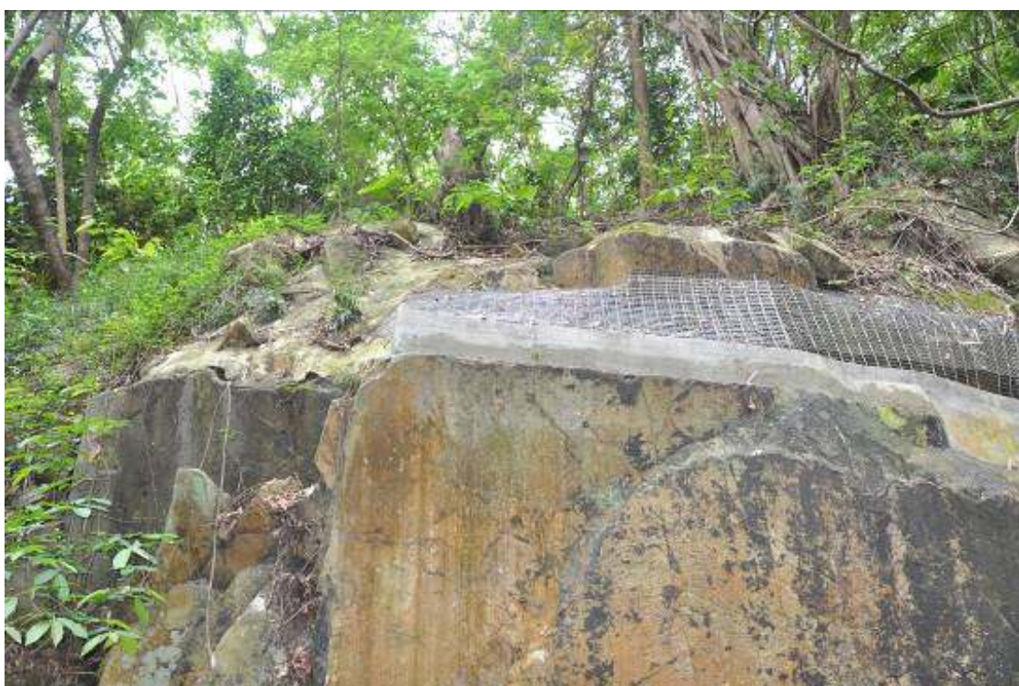
Figure 96. View of the cement barrier and mesh place above the engravings, and of the capping covering the upper parts of the stream walls.
