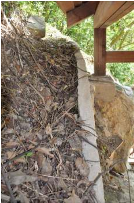
Figure 8. Accumulation of earth and leaves on the channel
