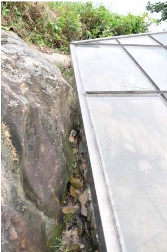
Figure 102. Detail of the area where water should be channelled away from the engravings, filled with soil and leaves, and visibly very damp
