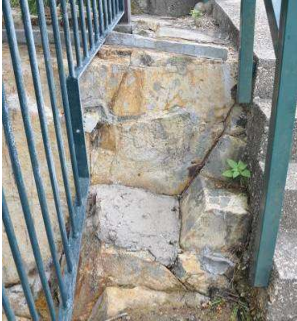
Figure 84. Detail of cement remains at the site, which should be removed.
