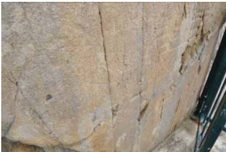
Figure 37. Unstable and partially detached fragment
