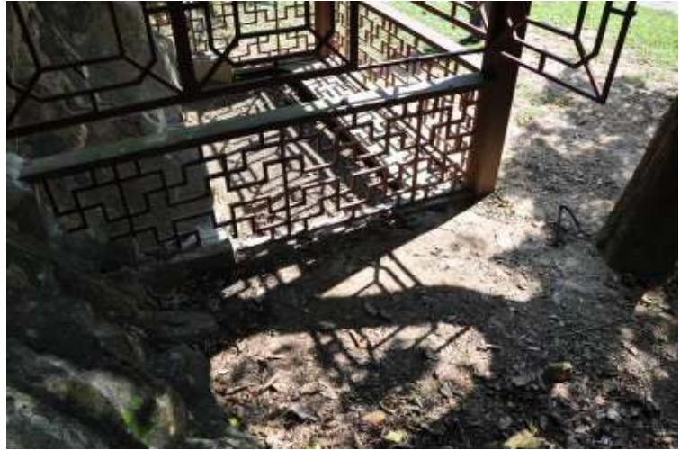
Figure 7. View of the area north of the shelter, where water is channelled. Note the higher level of the ground in this area, in comparison to ground level inside of the shelter.
