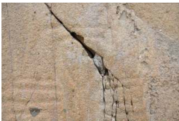
Figure 35. Detail of an apparently dry root inside a crack
