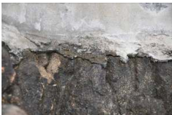
Figure 47. Detail of the poor contact between the cement and the granite
