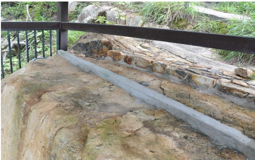
Water diversion dam above the Rock Carving
