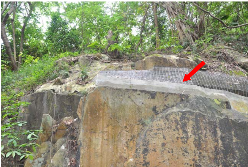
Water diversion dam with mesh placed above the Rock Carvings
