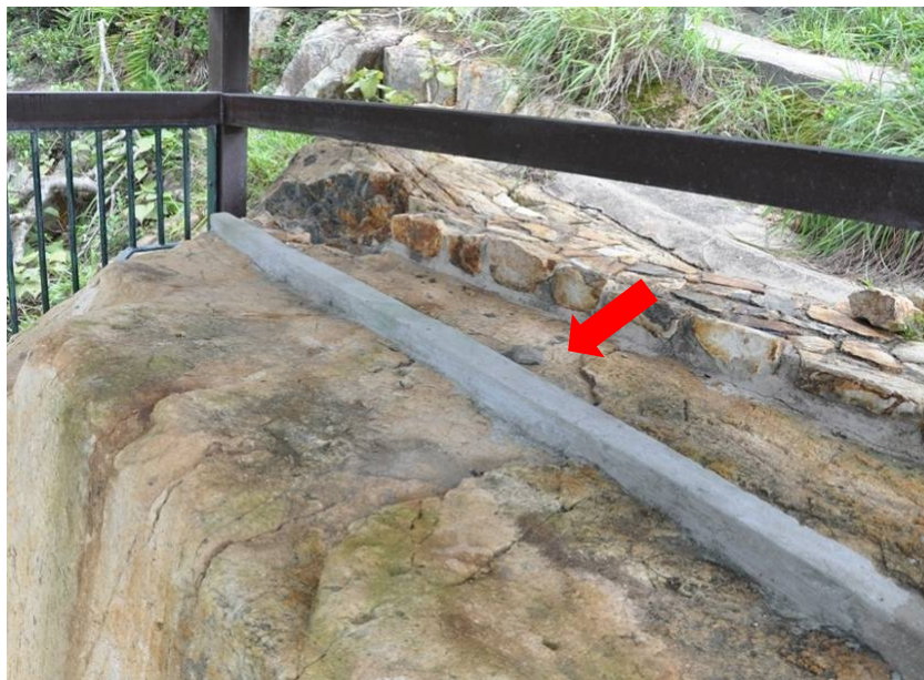
Photo 1: Water diversion dam above the Rock Carving
