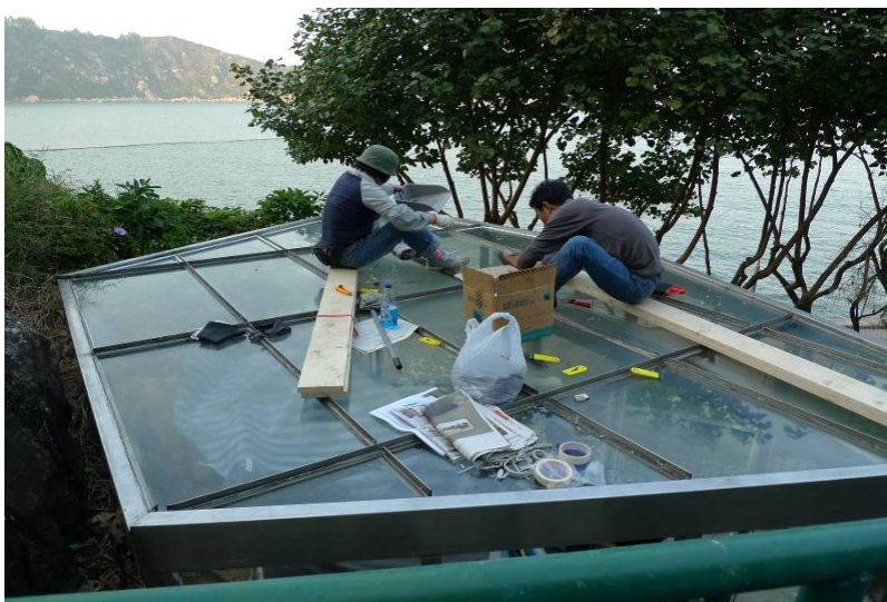
Photo 9: Re-seal of the glass roof to stop the water leakage
