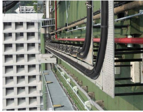
(LEFT) EXISTING CONDITION ON EAST WING ARE LAID WITH MULTIPLE SERVICE PIPES AND DUCTS EXPOSED TO NEIGHBORING BUILDINGS
