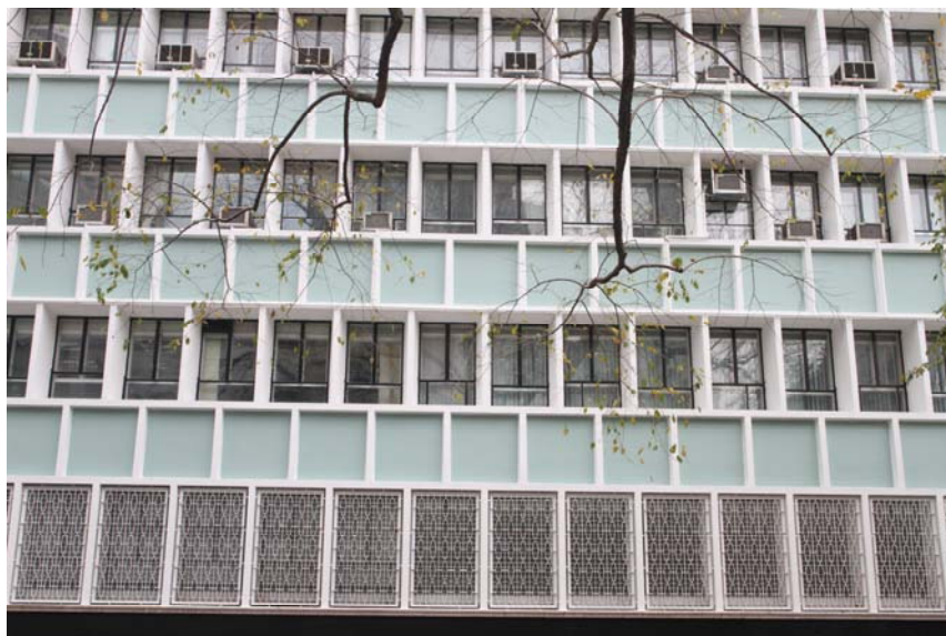
Fig. 17 Windows of the Main Wing. All windows of the CGO site are in Universal Crittall Style with a simple frame and proportional light design
