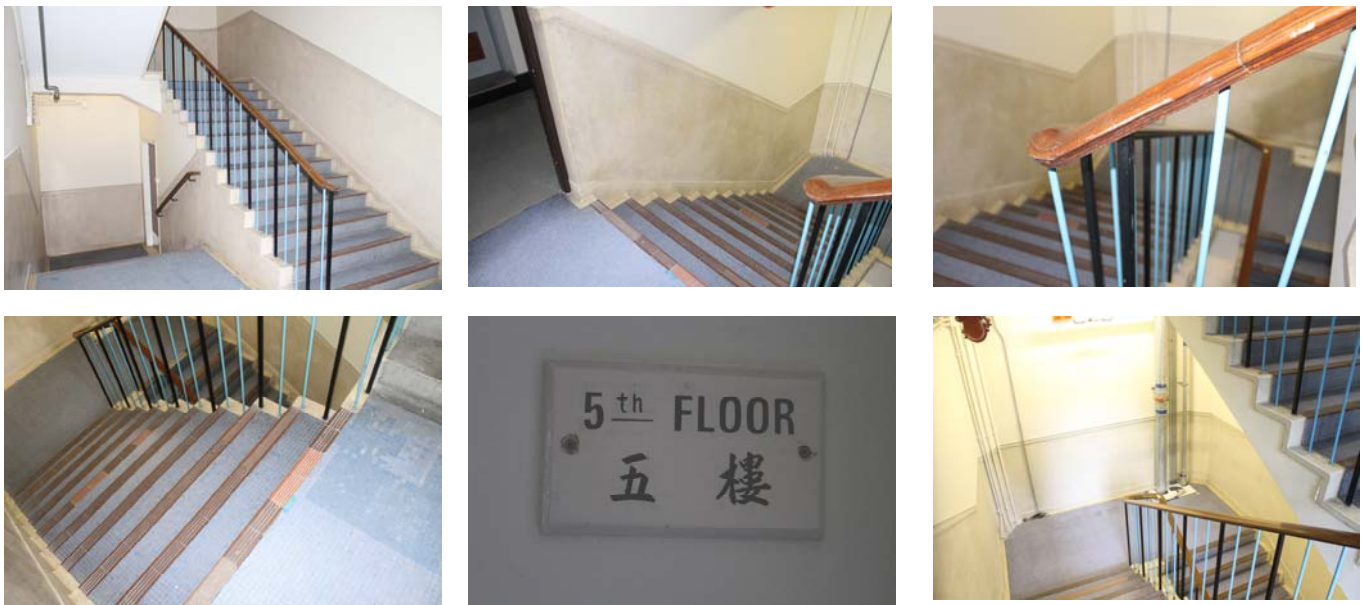
Fig. 79-84 (Left to right, top to bottom) The East Wing behind the lift lobby preserved much of its features including the terrazzo finishes on dado levels (Fig.80), the metal railing with timber handrail (Fig. 81), blue mosaic tiles (Fig. 82), old floor signage board (Fig. 83) and ceiling moulding. However, later ductworks have found penetrating the floors which visually distorted the outlook of the stairs.
