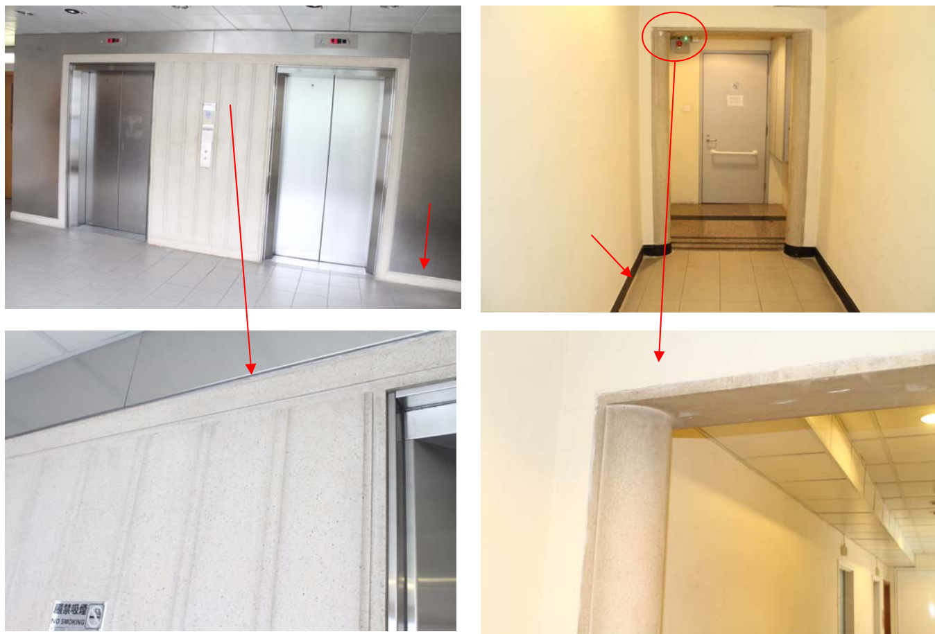
Fig. 75-78 (Left to right, top to bottom) show the original terrazzo finish found in the floor lobby area. They are preserved respectively on the lift surround (Fig. 75) with vertical fluting pattern,(Fig. 77) ,wall footings (pointed in Fig. 75 – 76) and the porch surround to the rear side toilets (Fig. 76, 78)
