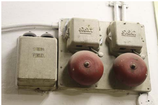
Fig. 133 (Top left) the meter located in B/F & Fig. 134 (Bottom left) the double-bell fire alarm system are old products manufactured by General Electronic Company (G.E.C.) from Britain. G.E.C. (Fig. 135, Top right) is a British-based company once being the world-pioneer enterprise in developing different kinds of electric products which make the invention of electricity enhance human life in great extent in 19 th & 20 th centuries. The brand was bought and renamed in 1999.
