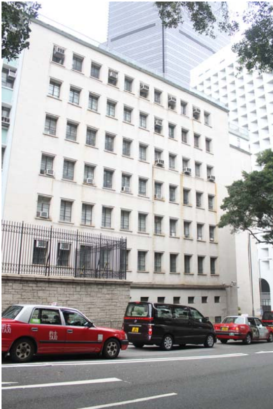
Fig. 24 (Left) and Fig. 25 (Right) showing the two-linked square tower design on the east side of the East Wing. The main entrance is design on the south junction between these 2 square tower blocks (Pointed in red). The additional floor on the top of right square tower is a much later additions done in 1970s with the original cornice flag pole demolished with marks remain. (pointed in black)
