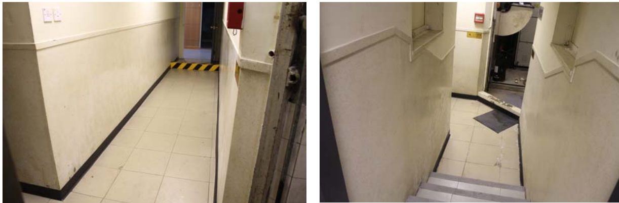
Fig. 112-113 (Left to right) The untouched terrazzo finishes at dado level and window sills located on the pathway next to the LG/F Plant Room.
