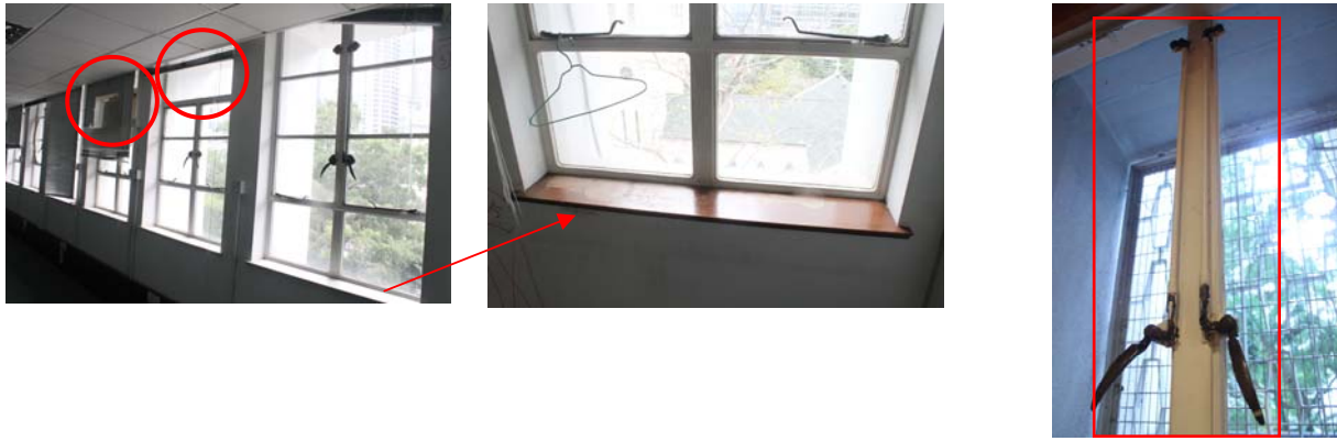
Fig. 100-102 (Left to right) show the Universal design of the East Wing windows. The design of the windows are in 8-light, alterations in later stage are found in part of windows which can be revisable. (Fig. 100 alteration with circles). The windows are bottomed by timber sills (Fig. 101) and locked in a vertical double-lock and single-handrail system (Fig. 102, squared)
