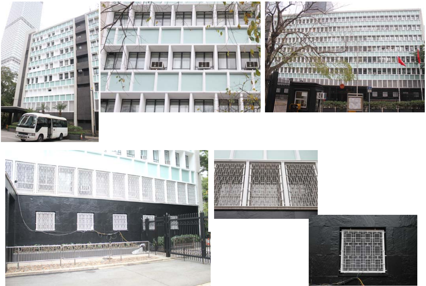
Fig. 42 – 47 (Left to right, top to bottom) The west elevation of the north annex block (Fig.42), the south old block (Fig.44) and the exposed concrete frame details (Fig. 43). Black-painted slate covered G/F (Fig.45) and the security grilles on 1/F (Fig.46) and on G/F (Fig.47) window openings.
