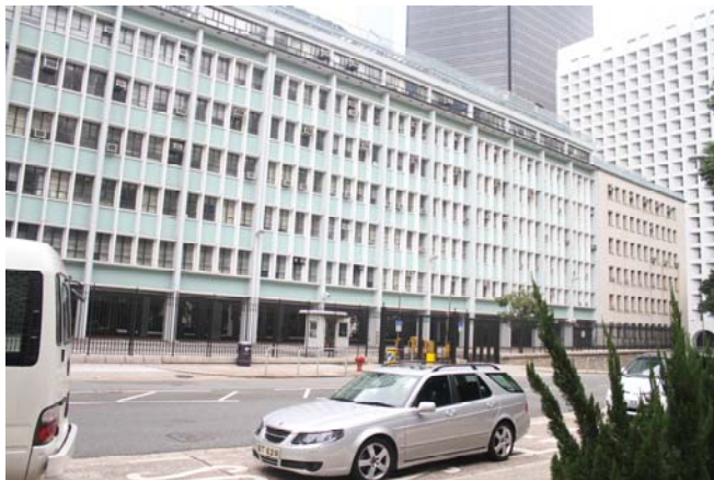
Fig. 18 (Left) showing the exposed concrete frame of central section and granite cladding right section of East Wing.
