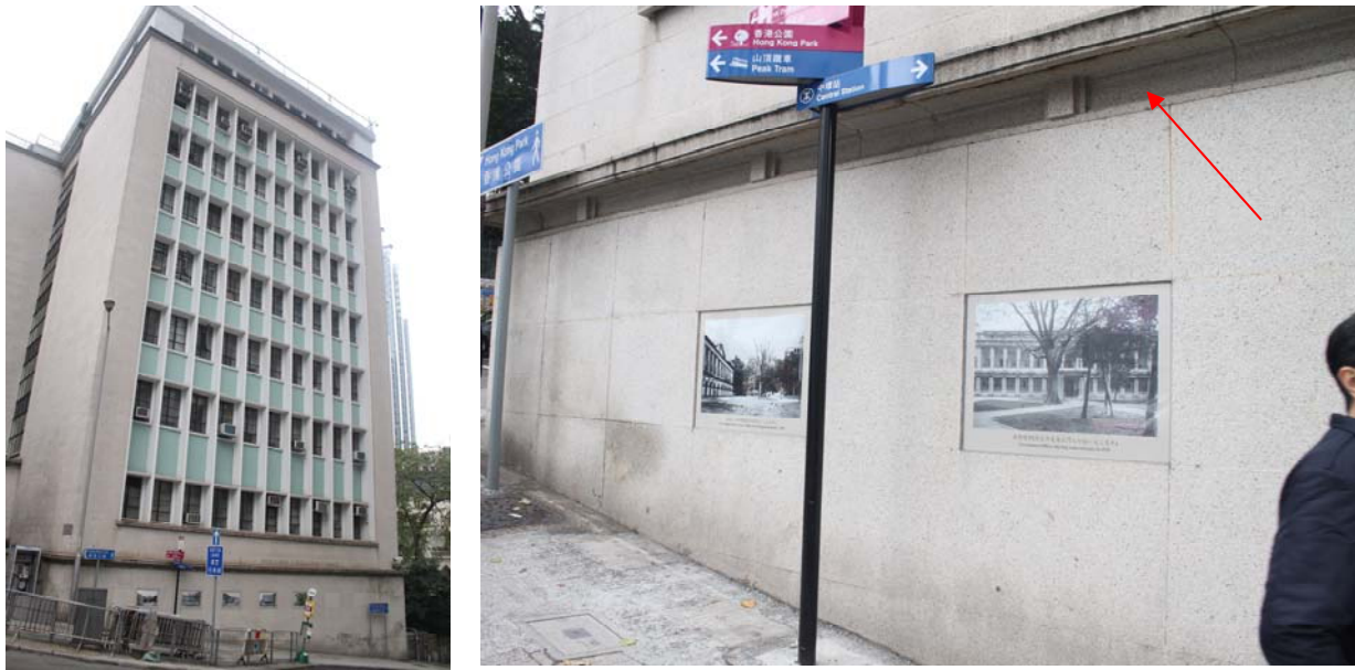
Fig. 38 (Left) & 39 (Right) show the mixture of exposed concrete frame with granite cladding surface design within one elevation. The basement of the block separated by an elaborated cornice (Pointed) was refurbished 2-3 years ago by inserting 5 glass frames with old photos of the CGO for public appreciation
