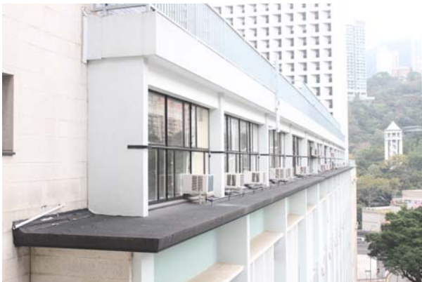
(Fig. 22, left) The additional floor added on the central part of East wing with its steel window frame design (Fig. 23, right).
