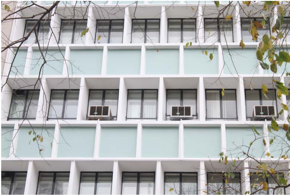
Fig. 15 The exposed concrete beam frame structures of East Wing alternate with rows of steel window and rows of green painted spandrel panels
