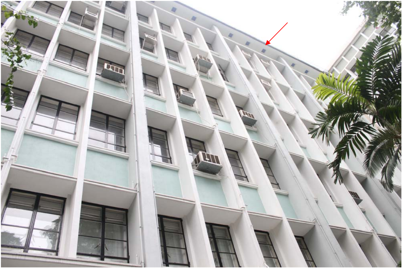
Fig. 21 A closer look to the central section of the East Wing on north elevation. The elevation with emphasis on vertical and horizontal elements divided the building into even bays. Each floor consists of a row of upper window with 8-light design, a projected window head and a shorter window sill. Under the window is a projected milky green-painted spandrel panels.
