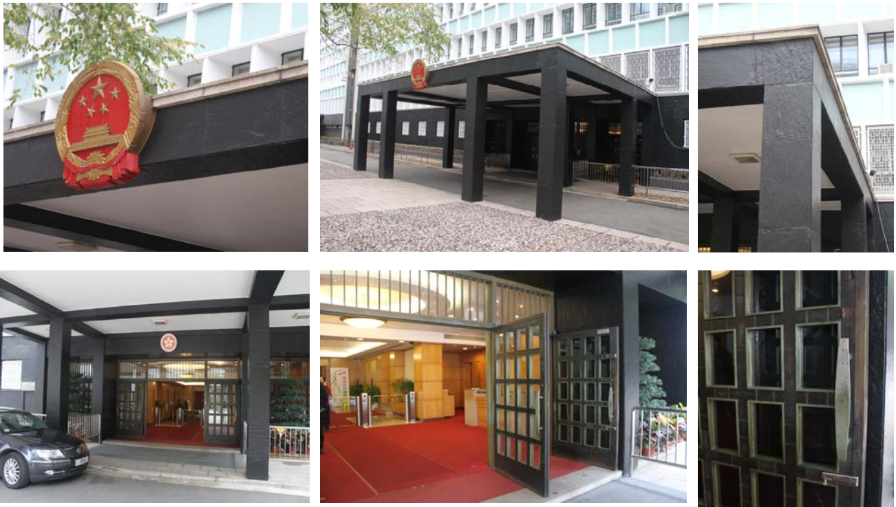
Fig. 48-53 (Left to right, top to bottom) The main entrance on the west elevation with detailed features including the PRC emblem on outer cornice level (Fig. 48), the canopy (Fig. 49), the slate surface (Fig. 50), the main entrance area (Fig. 51), the bronze entrance gates (Fig. 52) & its details (Fig. 53)
