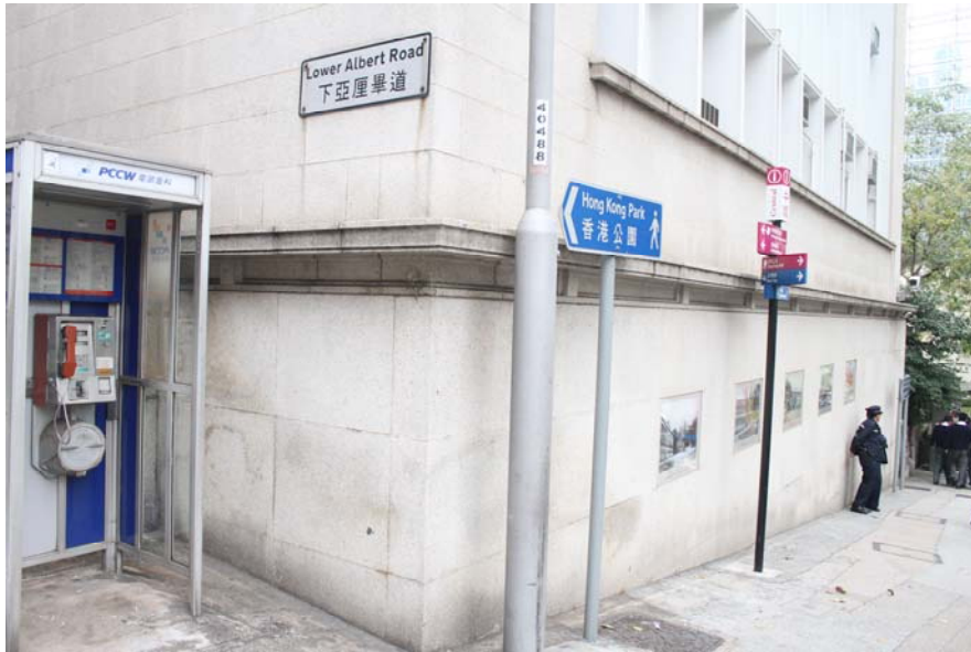
Fig. 16 The granite surface of the whole site is usually done with exposed surface without paint
