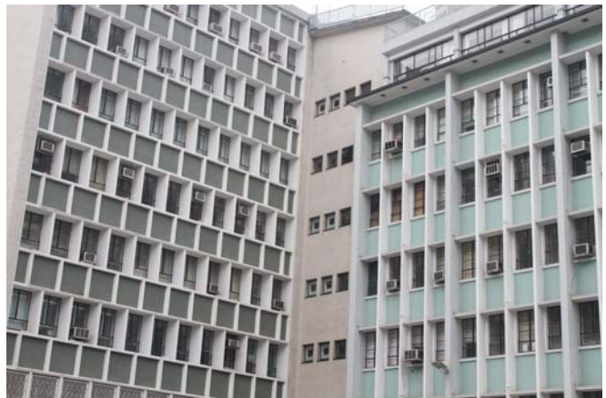
Fig. 18 (Left) showing the exposed concrete frame of central section and granite cladding right section of East Wing.
