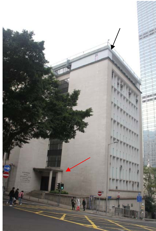
Fig. 24 (Left) and Fig. 25 (Right) showing the two-linked square tower design on the east side of the East Wing. The main entrance is design on the south junction between these 2 square tower blocks (Pointed in red). The additional floor on the top of right square tower is a much later additions done in 1970s with the original cornice flag pole demolished with marks remain. (pointed in black)
