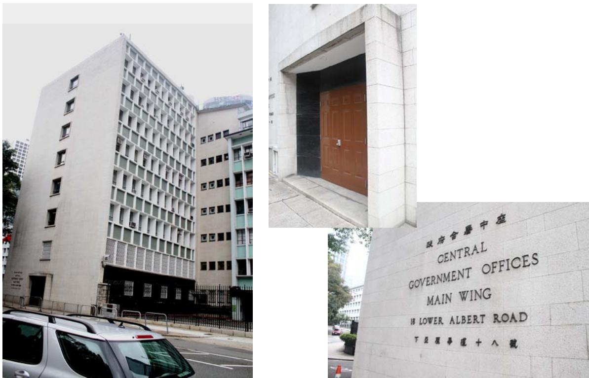
Fig. 54-56 (Left to right) The south elevation of the Main Wing. It is the only Main Wing surface solely with granite cladding. Distinct features include the granite porch old public entrance (Fig. 55) and the name of the building affixed on its left (Fig. 56).
