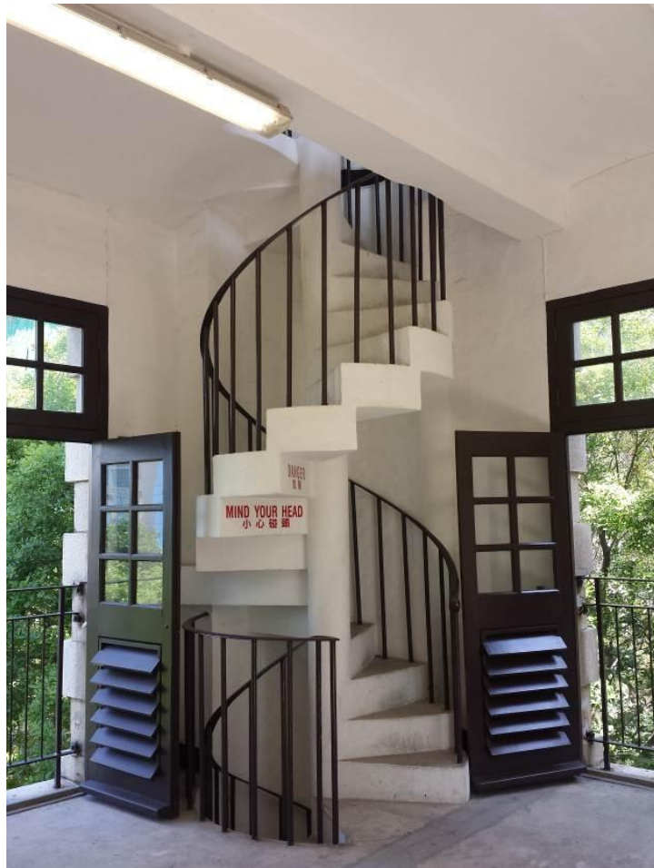
Concrete and steel spiral staircase on 1/F
