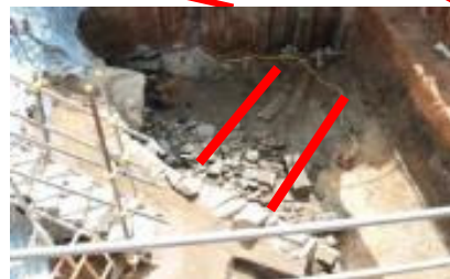
Stone footpath and stone structure which forms the riverbanks of the former Ma Tau Chung (Preserved in-situ)
