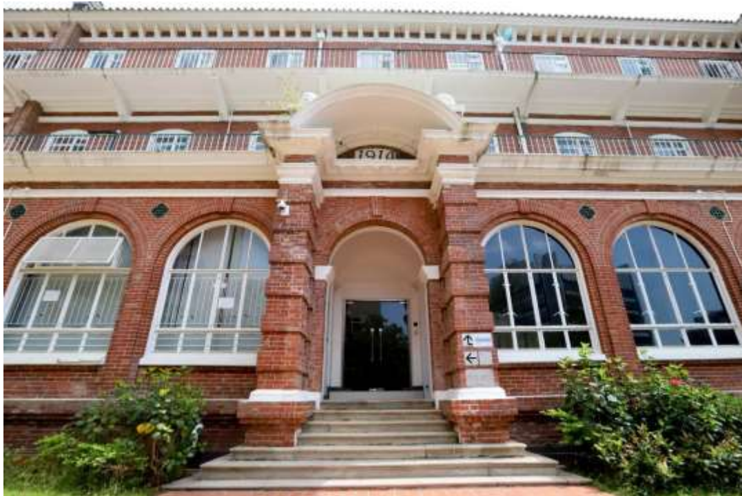
Rusticated brick piers and an elaborate shaped portico at the front façade
