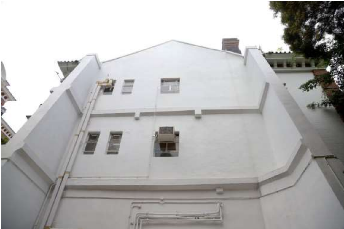
Two buttresses were erected at the collapsed portion after the severe landslide in 1966
