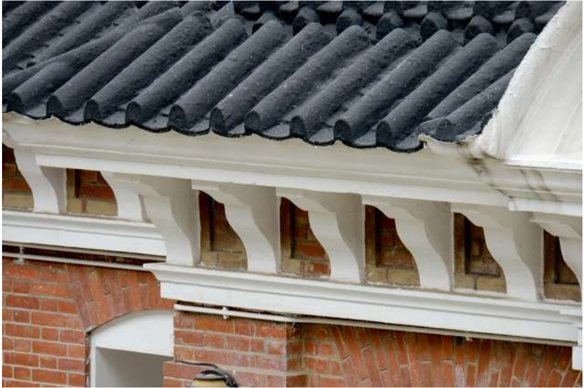
The roof eaves with numerous supporting brackets as a design feature, and a moulded cornice underneath
