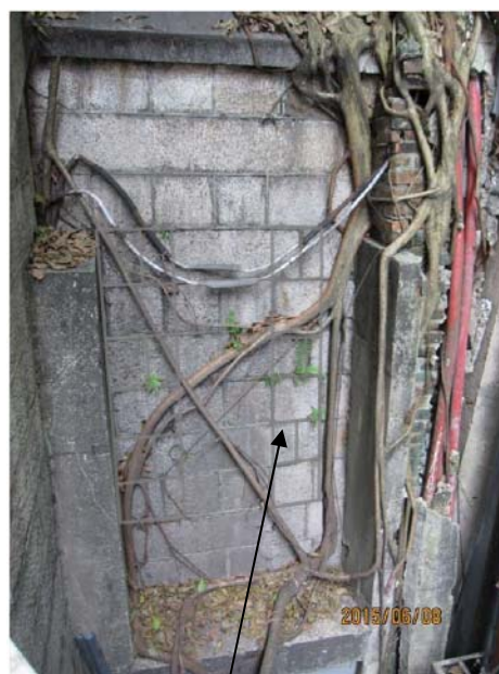
Vertical Recessed Soil Nail Beam Covered with Existing Masonry Blocks
