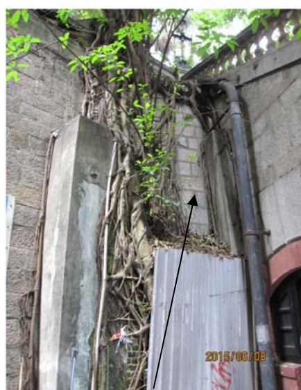
Vertical Recessed Soil Nail Beam Covered with Existing Masonry Blocks
