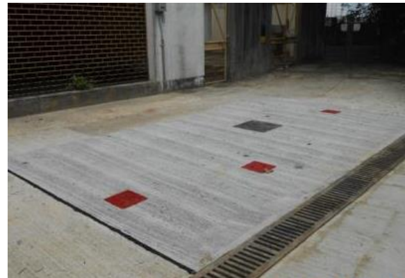
Photos 1 and 2 – Showing the Equipment Arrangement Installed in the Chamber and the Ground Surface Reinstatement after the Construction (approximate size: 1.5 – 3m wide x 1.5 – 5 m long x 2 – 4m deep)
