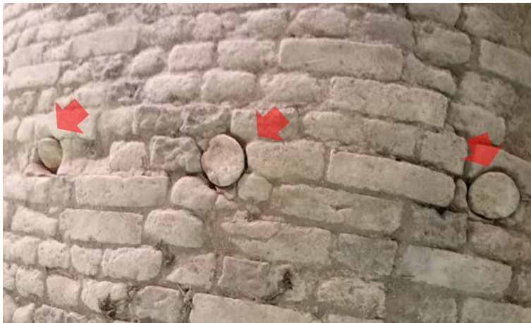
Fig. 19. Stroke holes on top of the fire chamber.
