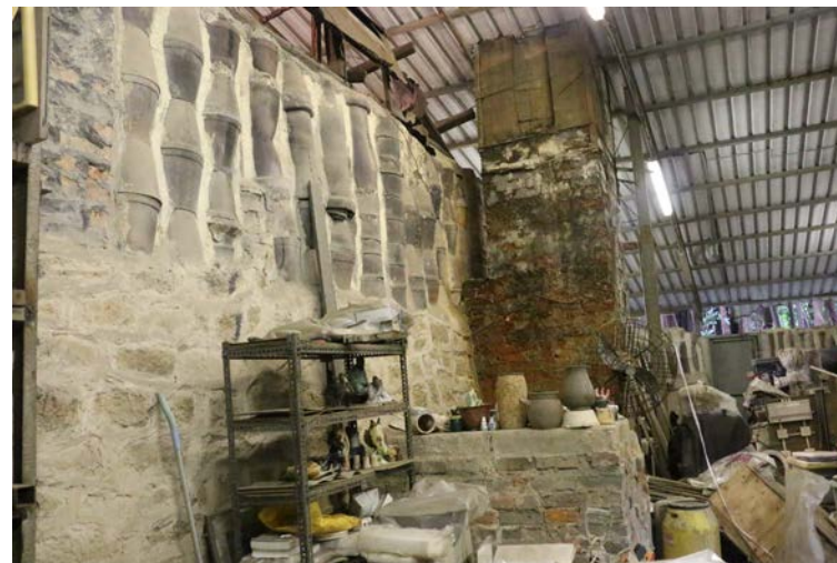
Fig. 22. The end wall above the end of the Ceramic Kiln made of pottery previously produced.
