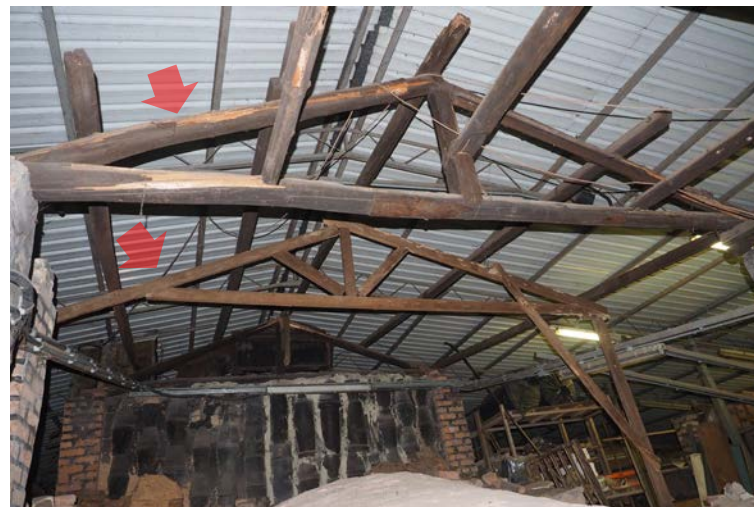
Fig. 26. Existing timber trusses for the original roof.
