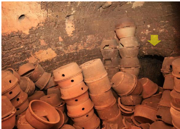
Fig. 21. The opening for the passage of smoke to the after burner at the end of the fire chamber, known as 喉嚨雞 [the throat of chicken] to the Shiwan people.
