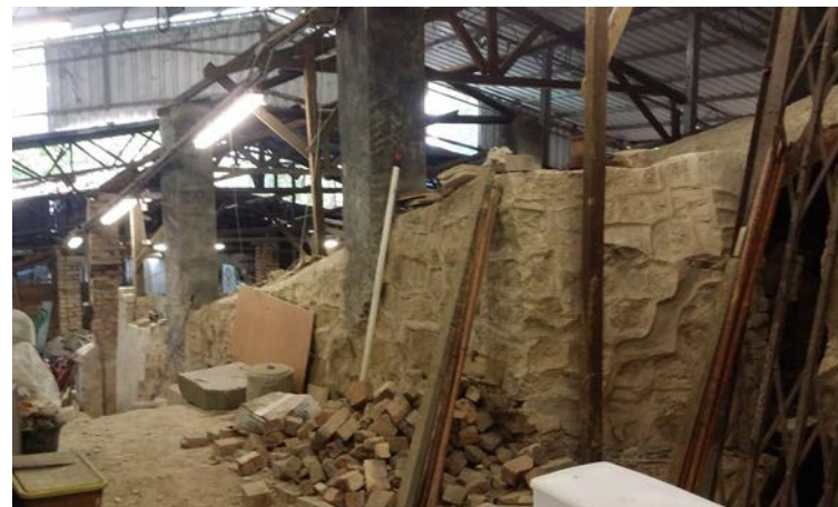
Fig. 16. Stone rubble wall on flanking both sides of the fire chamber.
