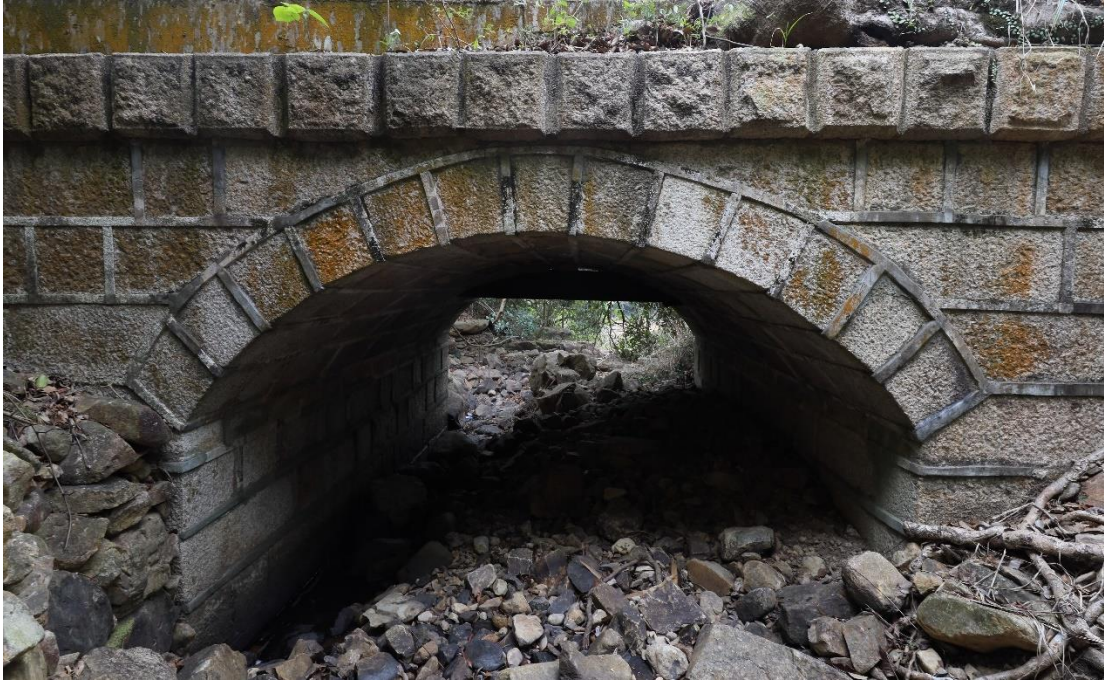
Close view of the Masonry Bridge. The Masonry Bridge is neatly finished with granite copings with chamfered margins and reticulated surfaces.
