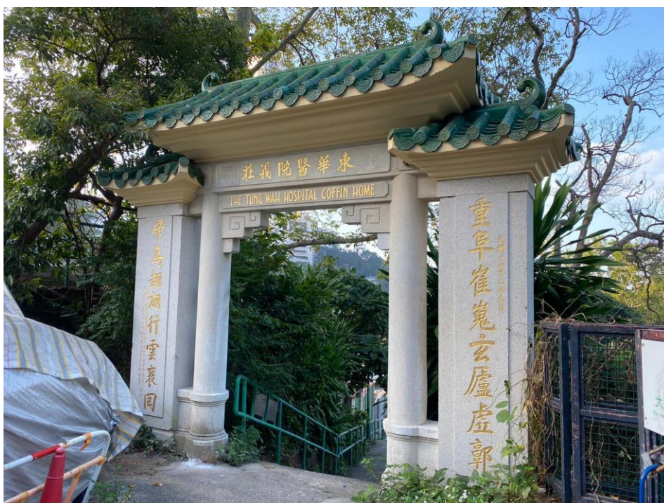
The coffin home's Chinese-style ceremonial pai lau (牌樓) near Victoria Road. It was built of granite and has a granolithic finish with green-glazed tiled roofs decorated with ridge-end ornaments and moulded cornices.
