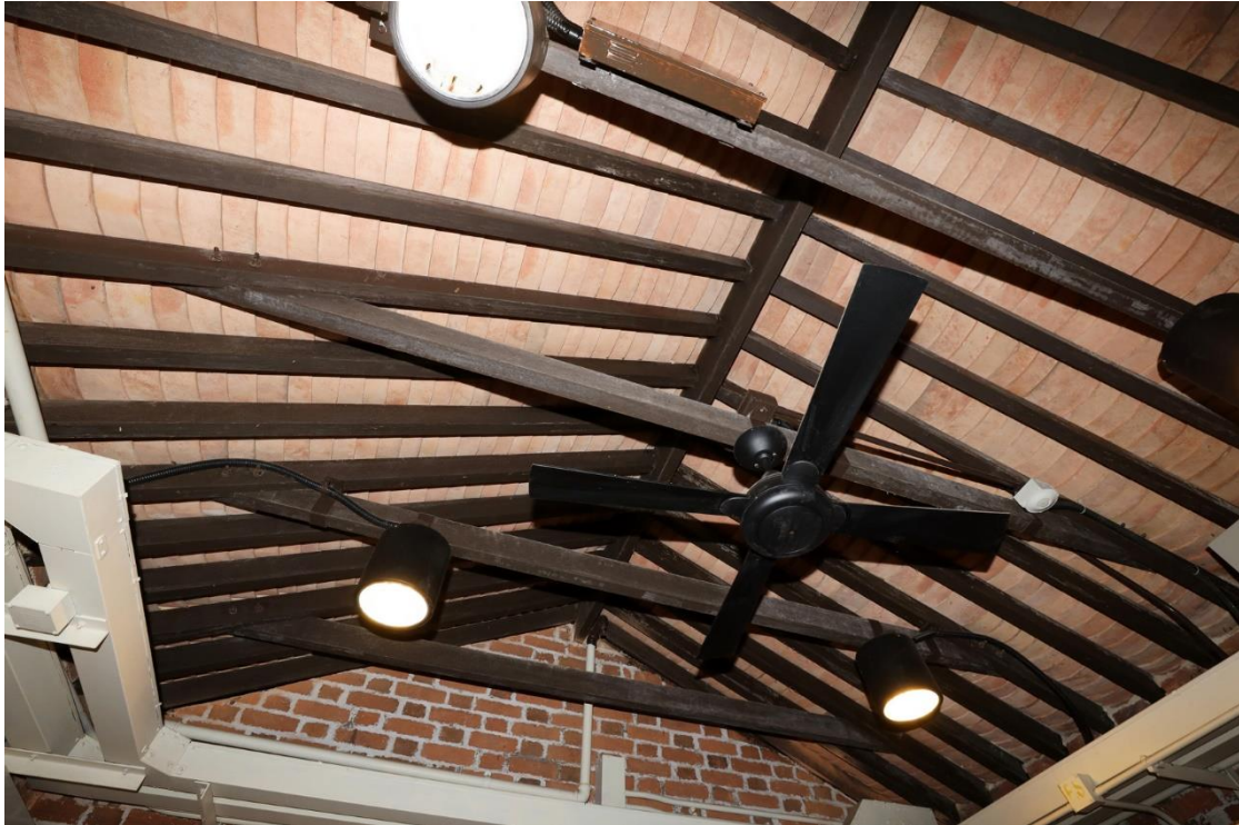
Chinese styled tiled pitched roofs supported by timber battens and purlins at Staff Quarters Block
