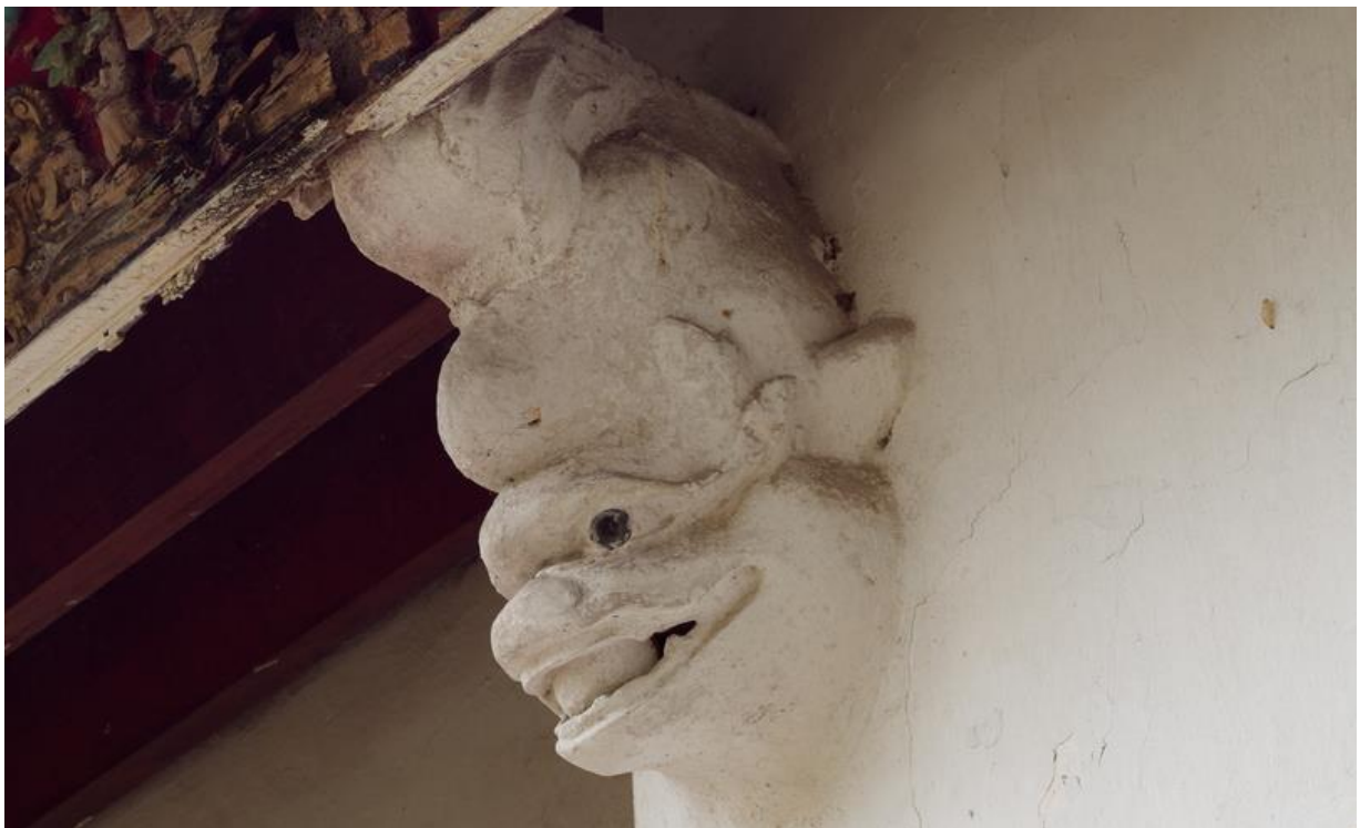
One of the two corbels plastered in the shape of dragonfish supporting the façade eaves
