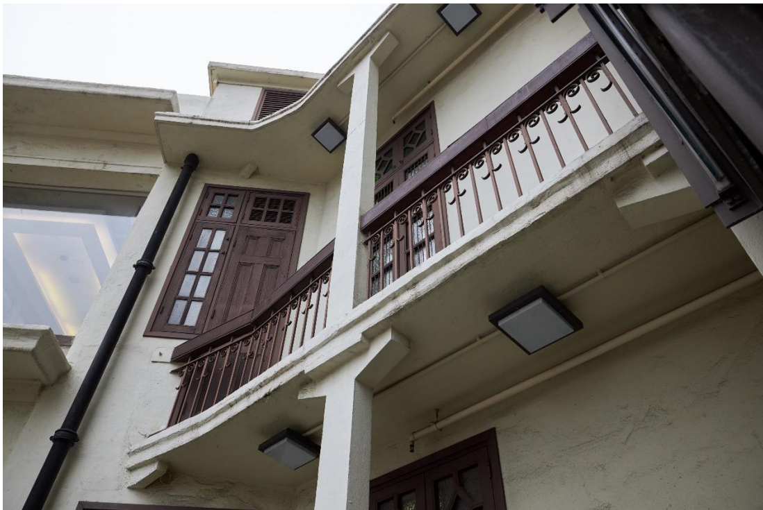
Rear verandah, supported by concrete beams, with the same pattern of railing.
