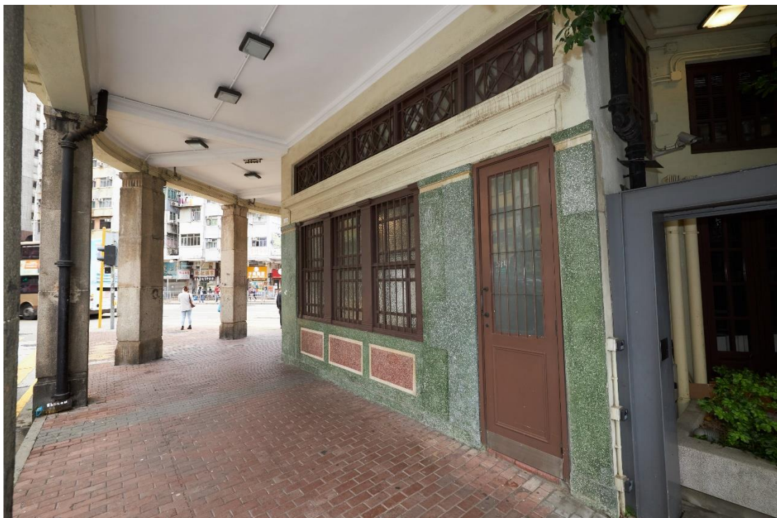
With granite columns supporting on the ground floor, the verandah extends over the public pavements forming arcades.
