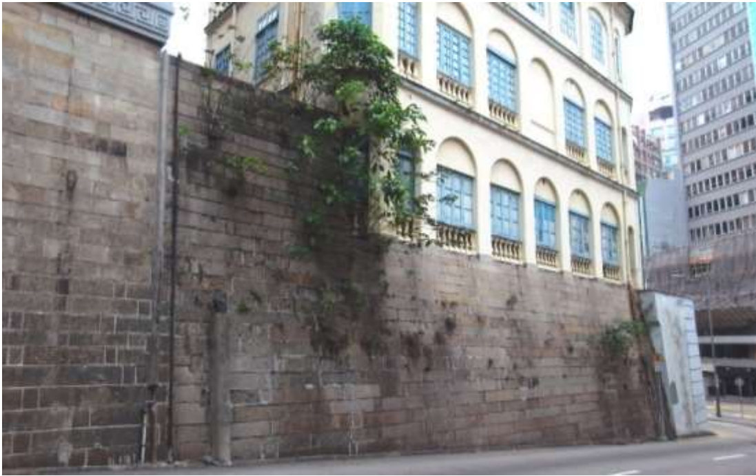
(a) Granite retaining wall on Arbuthnot Road
