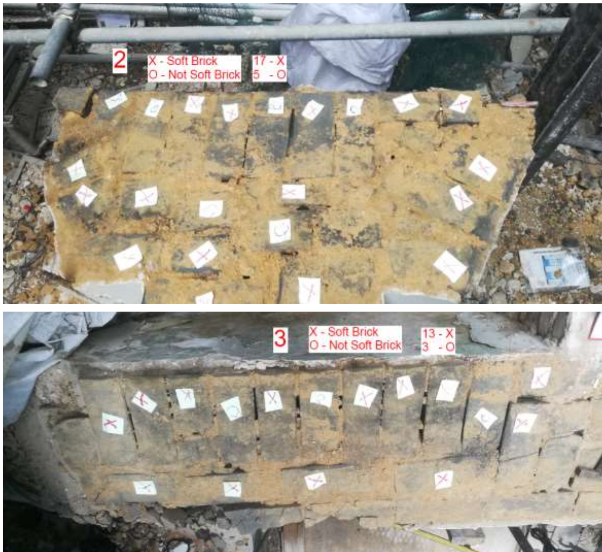
Figure 11 – (b) Approximately 75% of the bricks in random locations were considered soft (“X” Soft brick; “O” Not soft brick)
