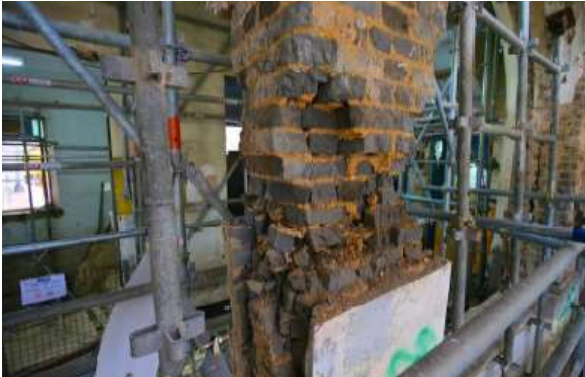
Before rebuilding (discovered on 27 September 2014) Extract from Appendix D2, 214A Repair Survey Report Revised, Building 04 – Married Inspectors, North Elevation, Central Police Station Hong Kong, Stonewest (HK)
