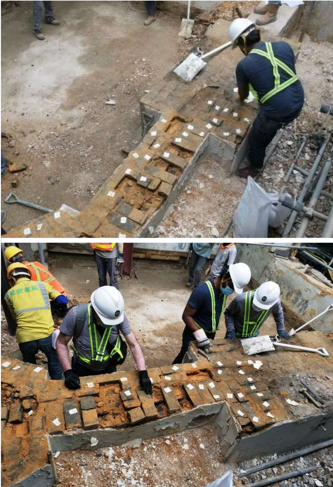
Figure 10 – Layer-by-layer inspection of brickwork during removal of the West Room by Purcell and Arup
