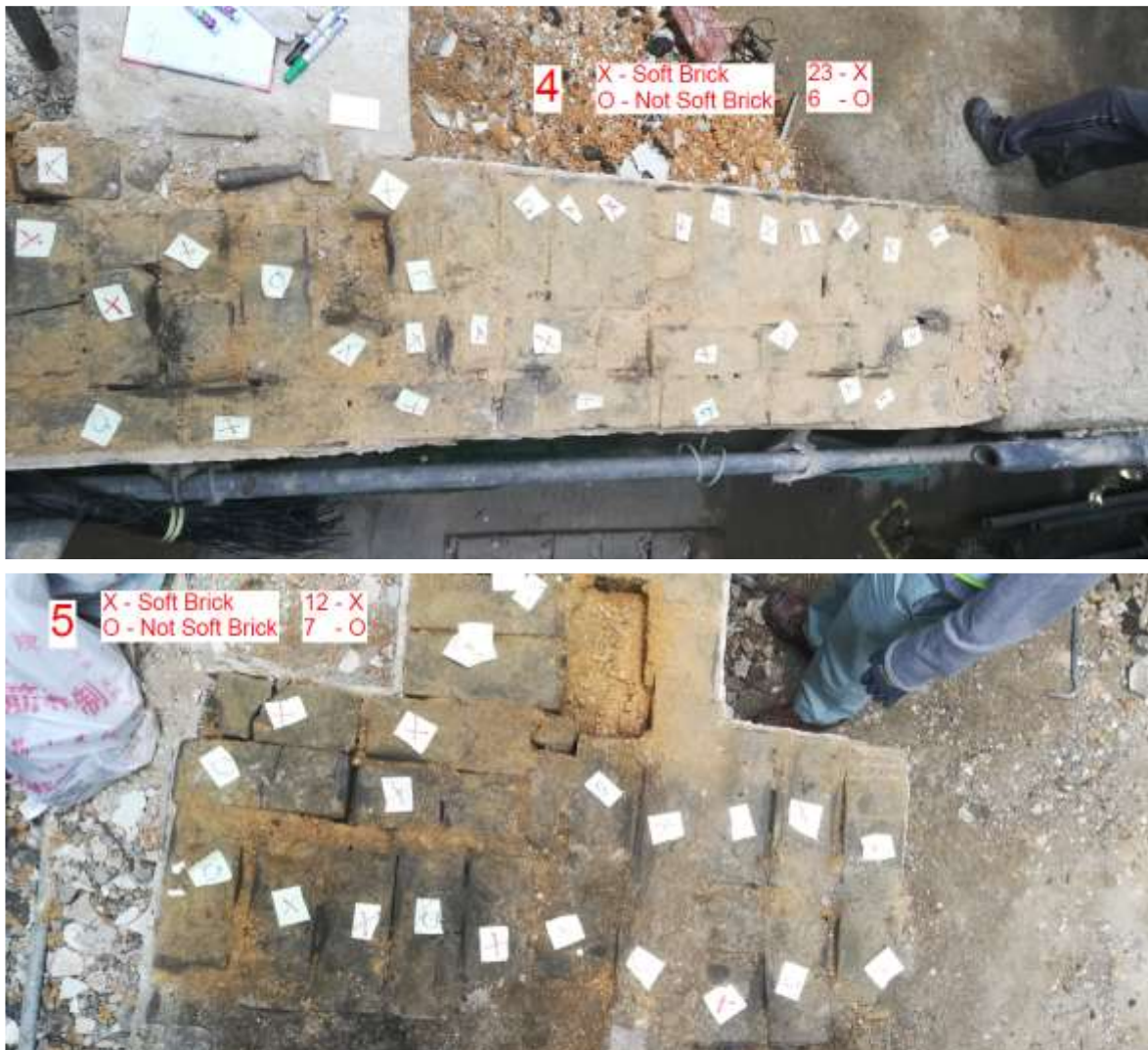
Figure 11 – (c) Approximately 75% of the bricks in random locations were considered soft (“X” Soft brick; “O” Not soft brick)
