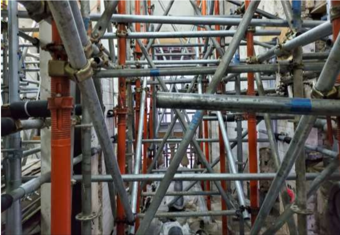
Figure 24 – Presence of densely installed propping (making it harder to undertake follow-on works safely)
