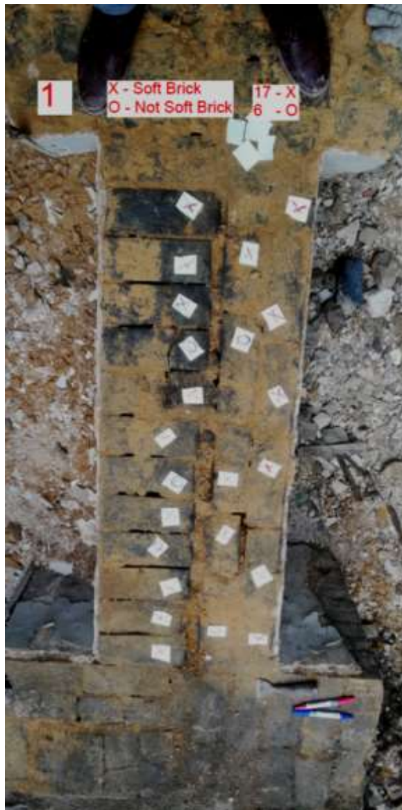
Figure 11 – (a) Approximately 75% of the bricks in random locations were considered soft (“X” Soft brick; “O” Not soft brick)
