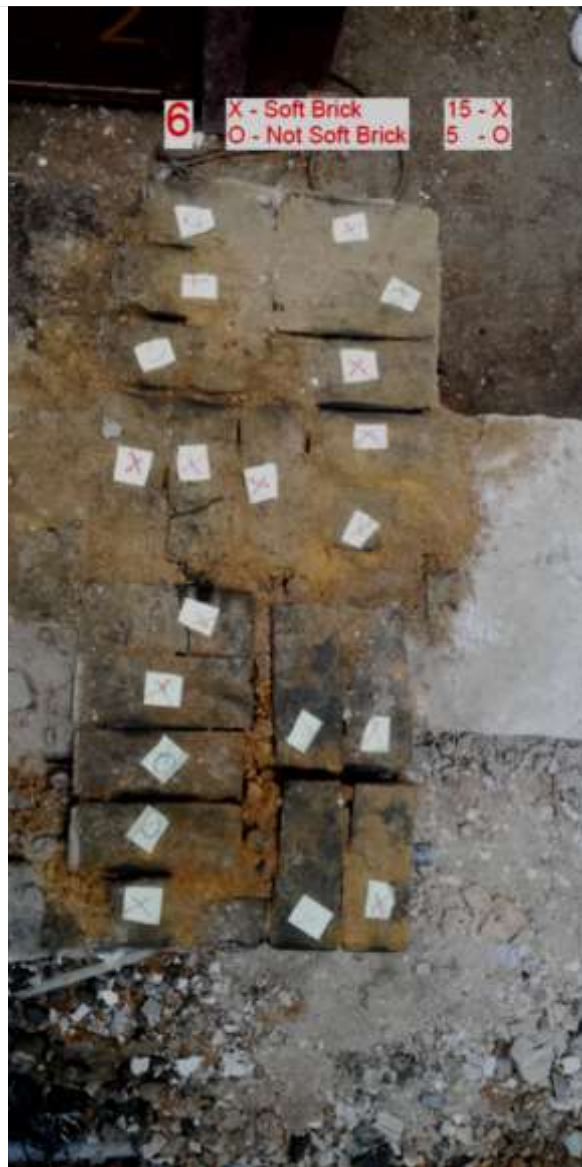
Figure 11 – (a) Approximately 75% of the bricks in random locations were considered soft (“X” Soft brick; “O” Not soft brick)
