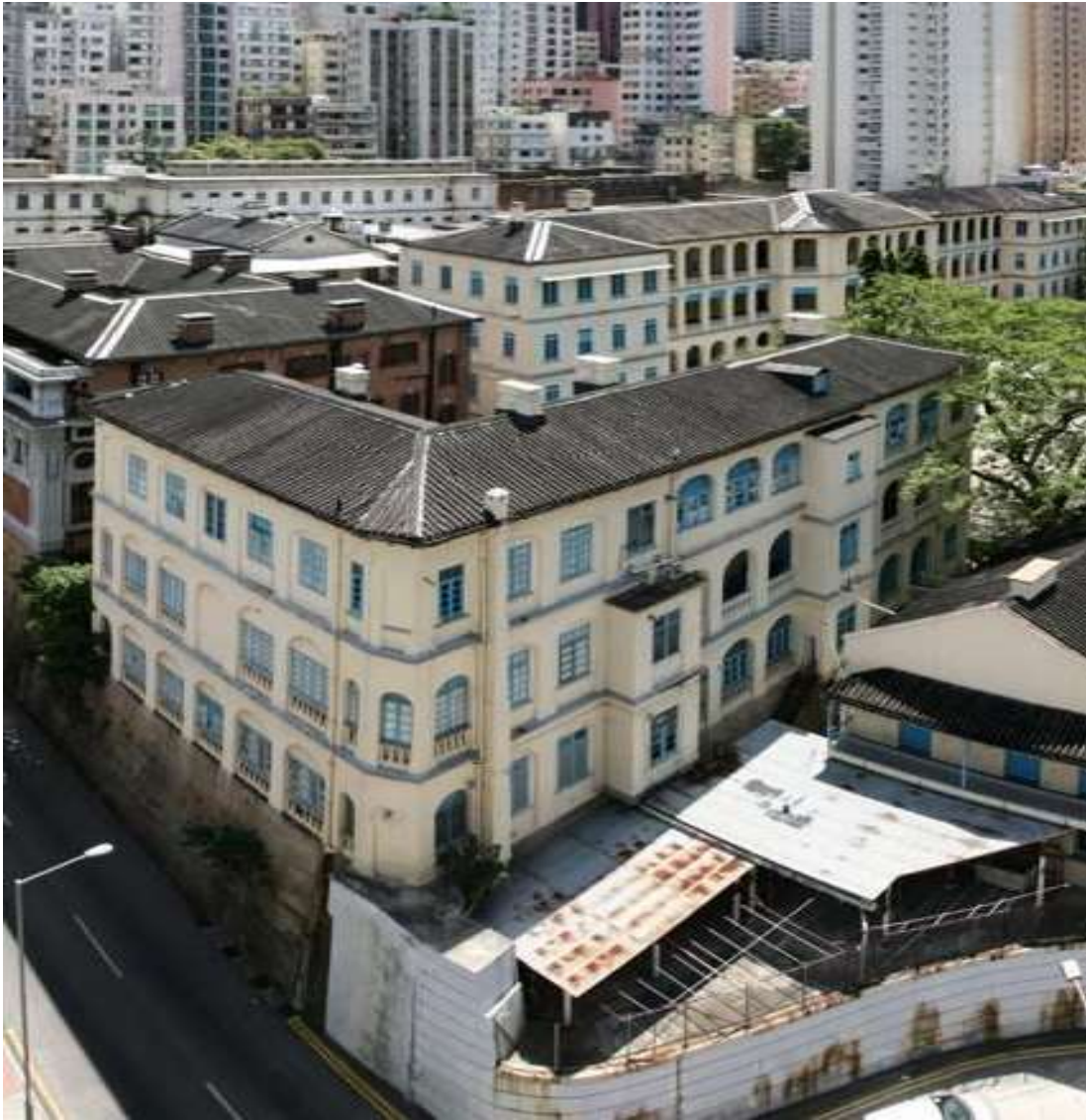
Figure 3 – Block 4 before partial collapse. The design provides relatively tall ceiling heights and large window openings to aid ventilation in the hot and humid climate of Hong Kong, resulting in large arched openings with brick piers in between on the north and east façades
