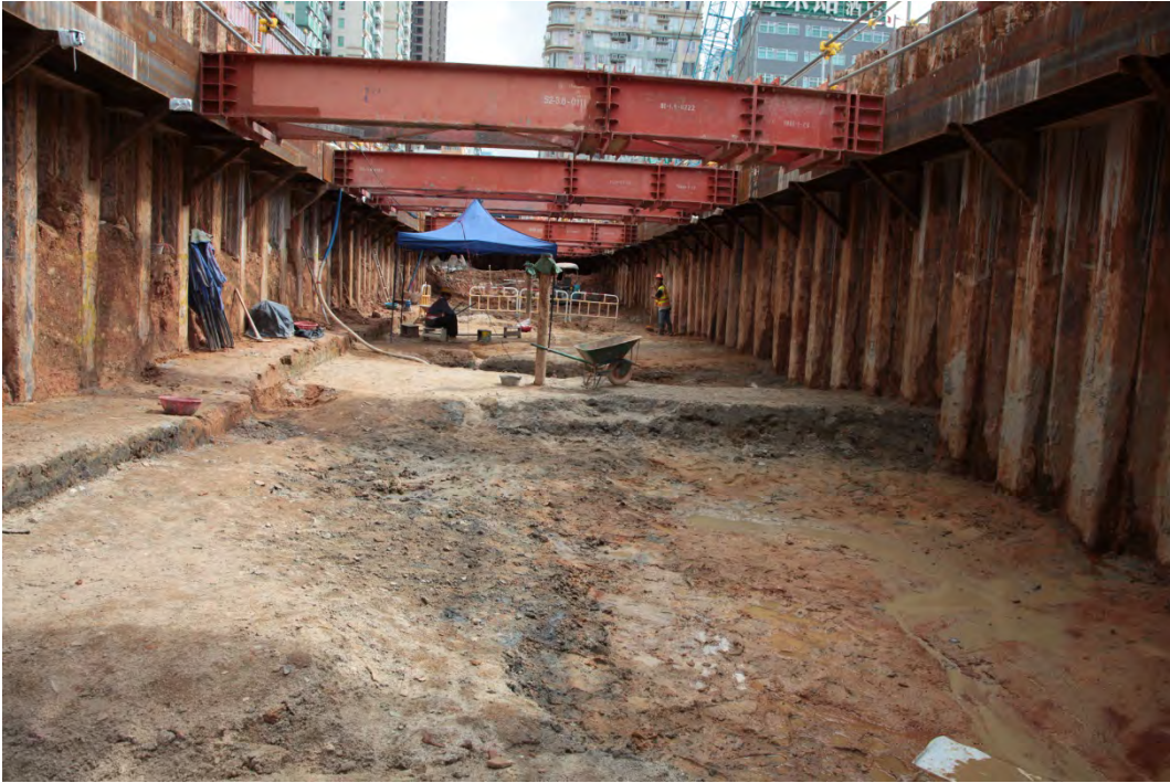
Present condition in Adit C(T2-T5) (from northeast to southwest)
