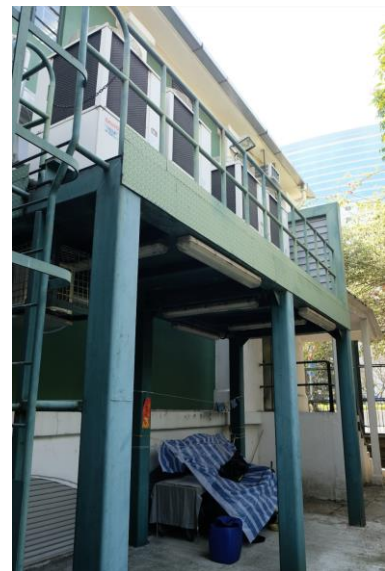
Figure 3-43 The metal structure supporting air-conditioning outdoor units.
