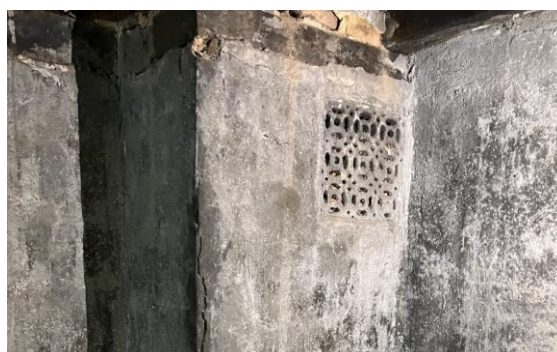
Figure 3-69 A cast iron air grille.
