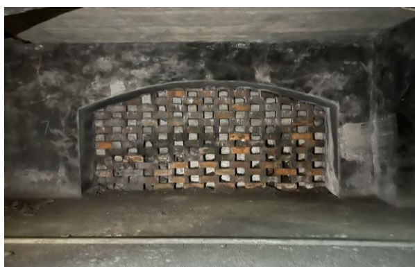
Figure 3-67 The honey-comb patterned brick screen wall.
