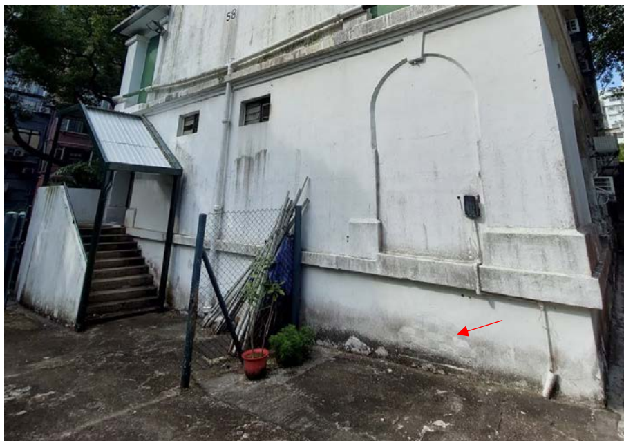
Figure 3-52 The base and middle sections of the east elevation and its attaching external staircase. Note that the original patterned brickworks of the arches at the base (arrowed) can still be traced even the arches are filled up currently.
