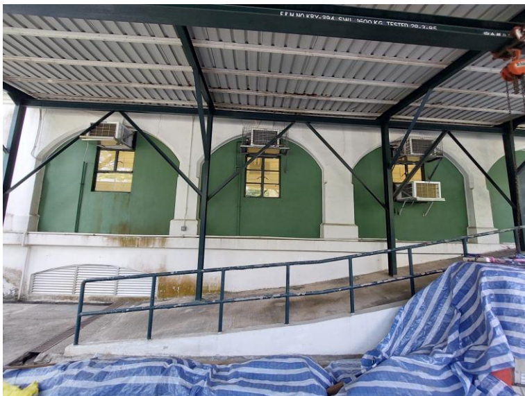
Figure 3-42 The new ramp on the north façade with the steel shed and pulley system above.
