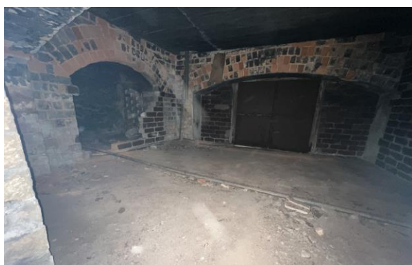
Figure 3-65 The segmental brick arches in basement.
