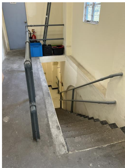
Figure 3-93 The cast iron posts and railings of the interior staircase.
