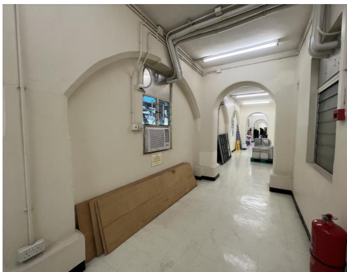
Figure 3-80 A cross arch (middle) and an arch on the internal side of the external wall (left) in G/F verandah.
