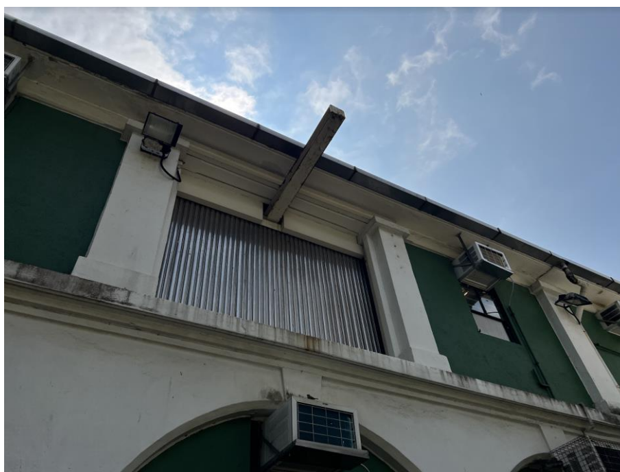
Figure 3-38 The later added hoist beam on the north façade.
