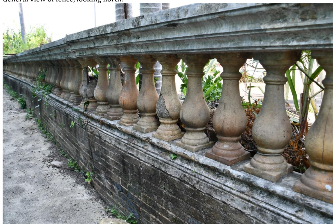
Dislocated and cracked fence, looking north.
