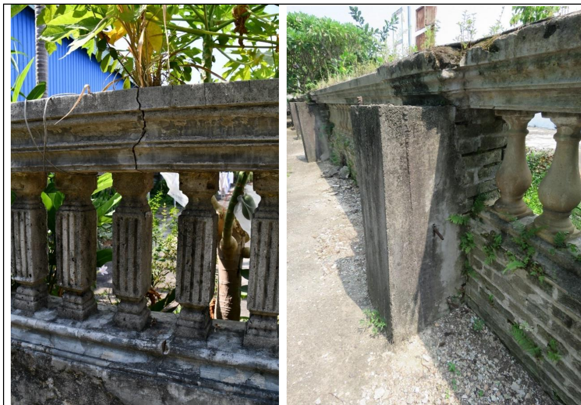
Close up of cracked section, looking northwest; and view of concrete buttresses; looking northeast
