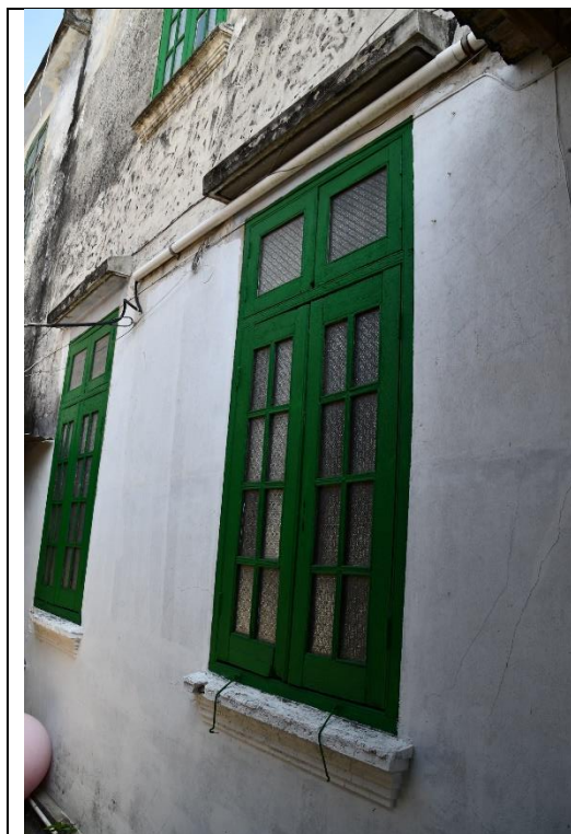
Window details: frosted glass panels set inside wooden frame
