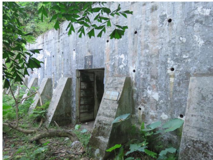
Bunker entrance location A, showing reinforced concrete terrace with buttresses, looking south. Note black paint above the entrance which shows the bunker number.
