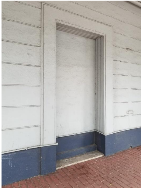
Fig.5.2.28 Both Stair 2 & 3 exit openings are blocked on ground floor, 2023 [by author]
