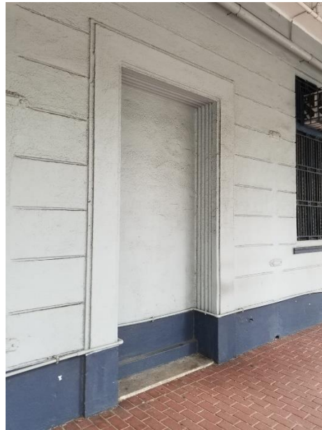
Fig.5.2.28 Both Stair 2 & 3 exit openings are blocked on ground floor, 2023 [by author]
