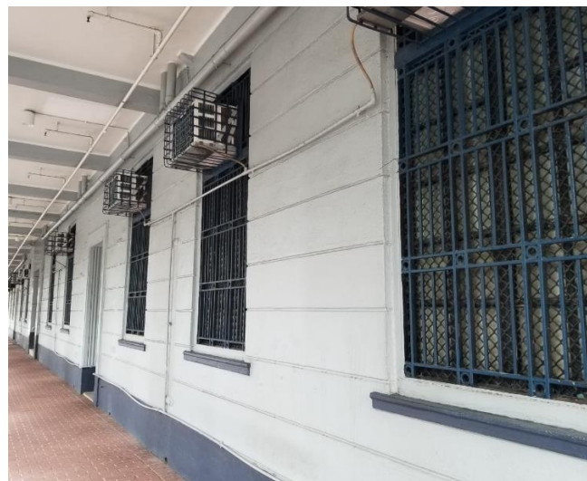
Fig.5.2.27 Security mesh and grill bar at windows 2023 [by author]
