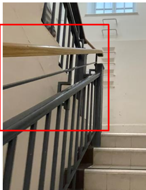
Fig.5.2.17 Stair railing extended, 2023 [ by author ]
