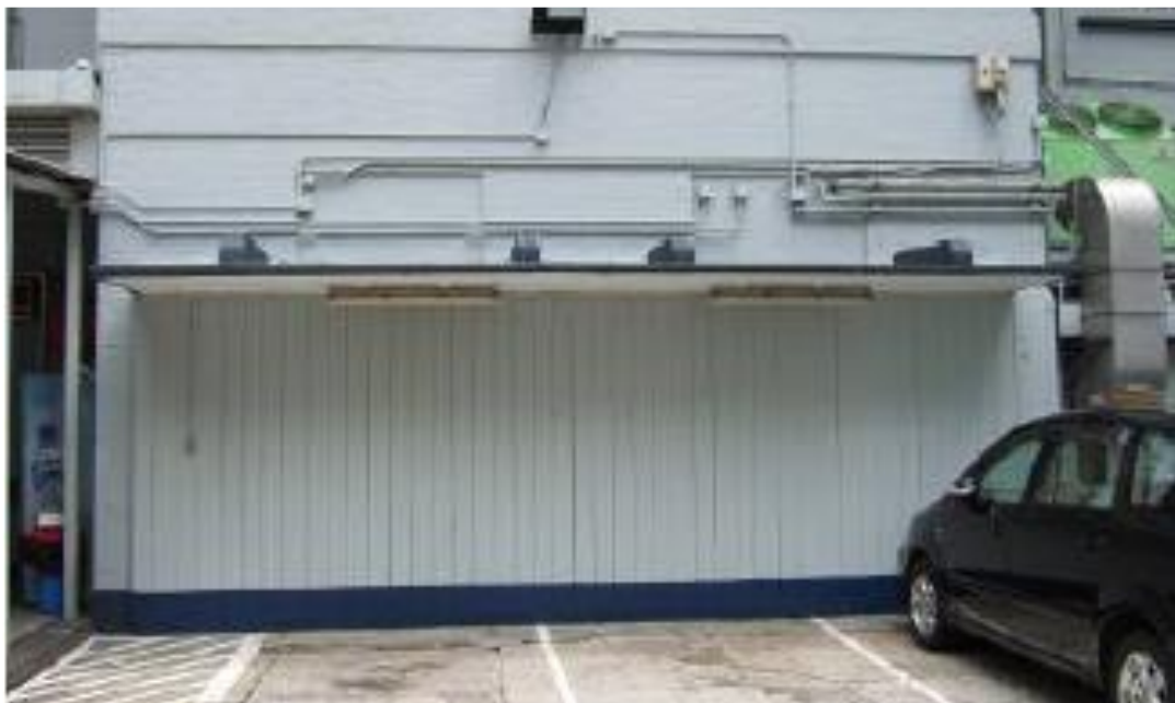
Fig.5.2.32 Centre wing wall & openings are blocked by wooden backstop which was further covered up by metal panels 2023 [by author]
