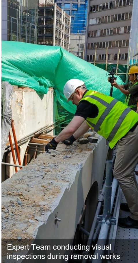
Figure 16 – Visual inspection during removal works, revealing copious evidence of substantial and widespread voids in brick vertical and horizontal joints
