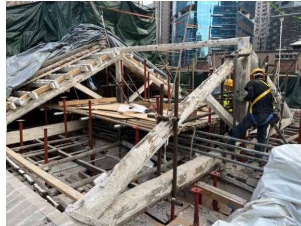
Removal of timber trusses
