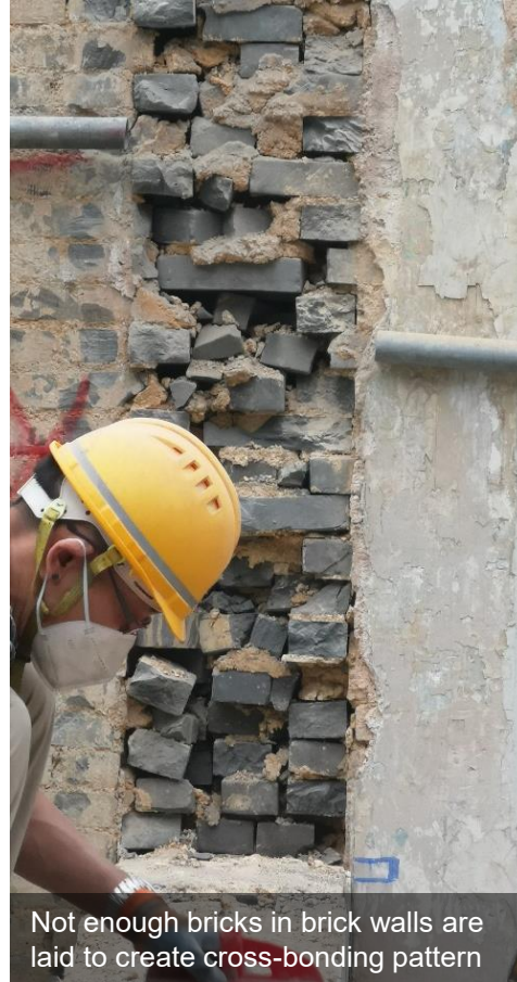
Figure 16 – Visual inspection during removal works, revealing copious evidence of substantial and widespread voids in brick vertical and horizontal joints
