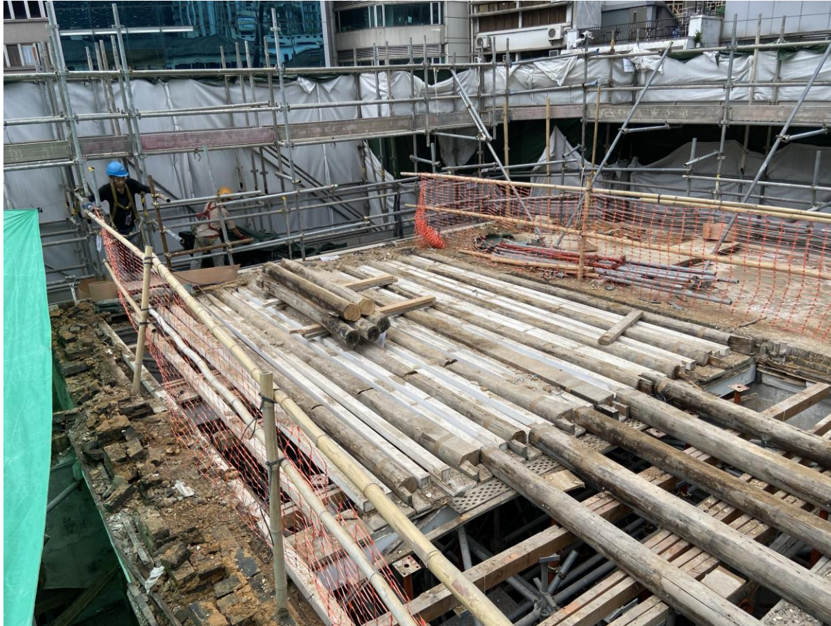
Figure 46 – Timber floor joists and new reinforcing steel beams (steel beams installed as part of revitalisation work in 2013-2016)
