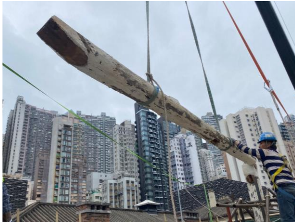
Removal of timber rafters
