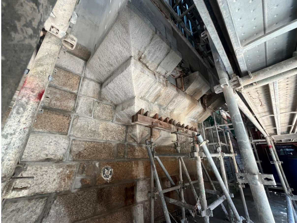
Figure 32 – Granite corbels of Block 4 supporting projecting bays
