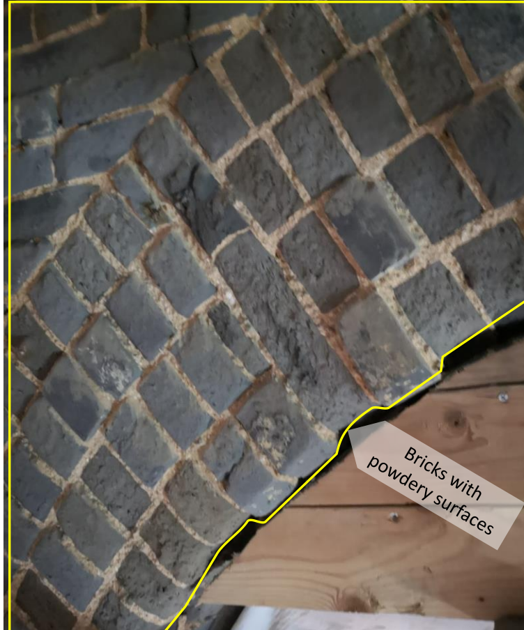
Figure 7 – Bricks with powdery surfaces seen in most areas of exposed brickwork (Location: Wall Zone W1 on 1/F)
