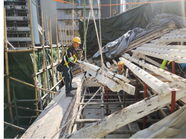
Removal of timber purlins
