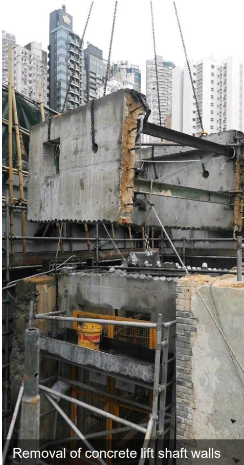
Figure 3 – Removal of unsafe building fabric at 2/F and 1/F of Block 4
