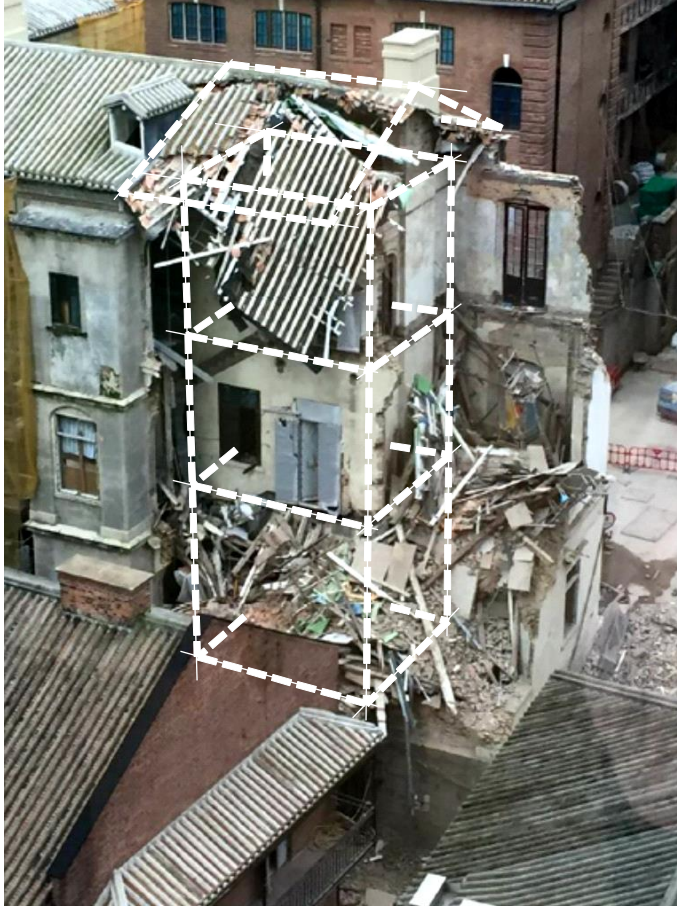
Figure 1 – Aerial views of partially collapsed Block 4 (North Wing) with extent of West Room indicated diagrammatically in broken lines
