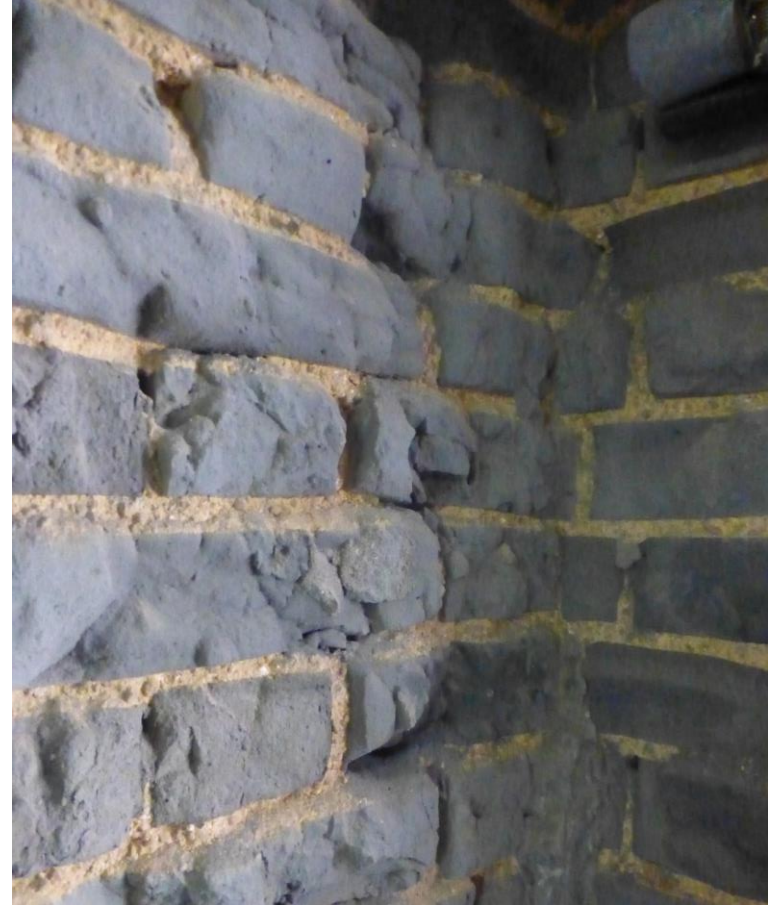
Figure 6 – Low-strength bricks seen in most areas of exposed brickwork (Location: Wall Zone W1 on 1/F)
