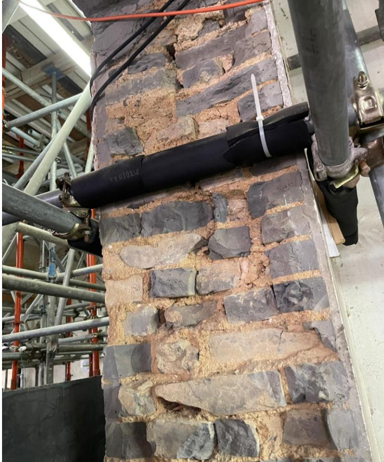
Figure 10 – (a) Poor bonding of brickwork, erratic in pattern and level (Location: Wall Zone W6 on G/F) (b) Through-thickness cracks in the west staircase portal (Location: Wall Zone W5 on 2/F)
