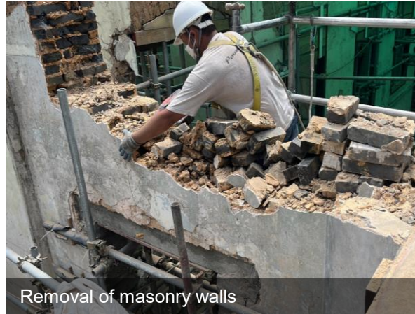
Figure 3 – Removal of unsafe building fabric at 2/F and 1/F of Block 4
