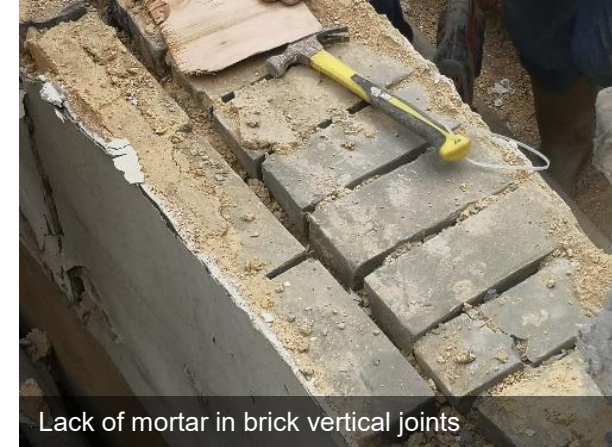
Figure 16 – Visual inspection during removal works, revealing copious evidence of substantial and widespread voids in brick vertical and horizontal joints
