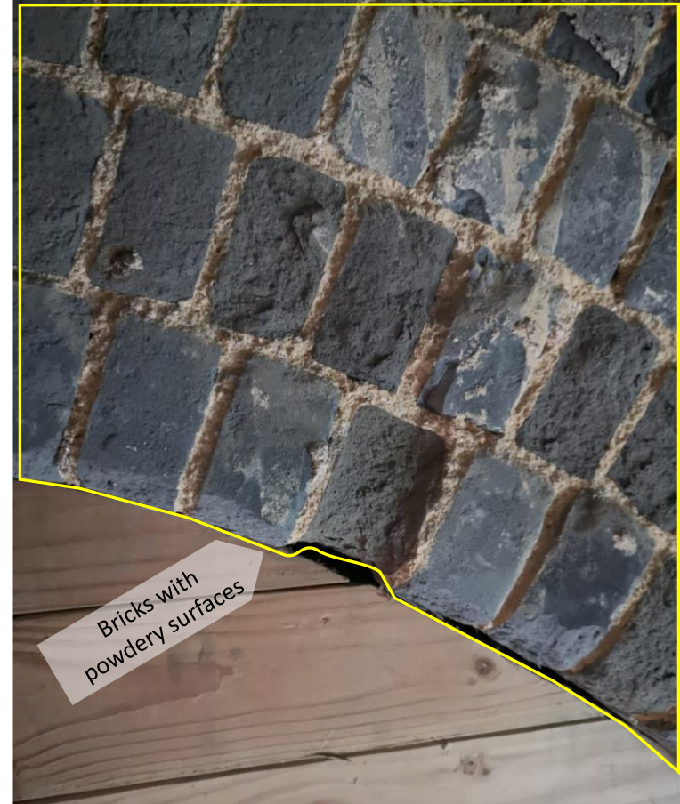
Figure 7 – Bricks with powdery surfaces seen in most areas of exposed brickwork (Location: Wall Zone W1 on 1/F)
