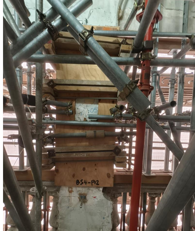
Figure 13 – (a) Cracks in brick pier noted after removal of window frame (Location: Wall Zone W4 on 1/F) (b) Failed pier stabilised by clamped timber boards (Location: Wall Zone W4 on 1/F)
