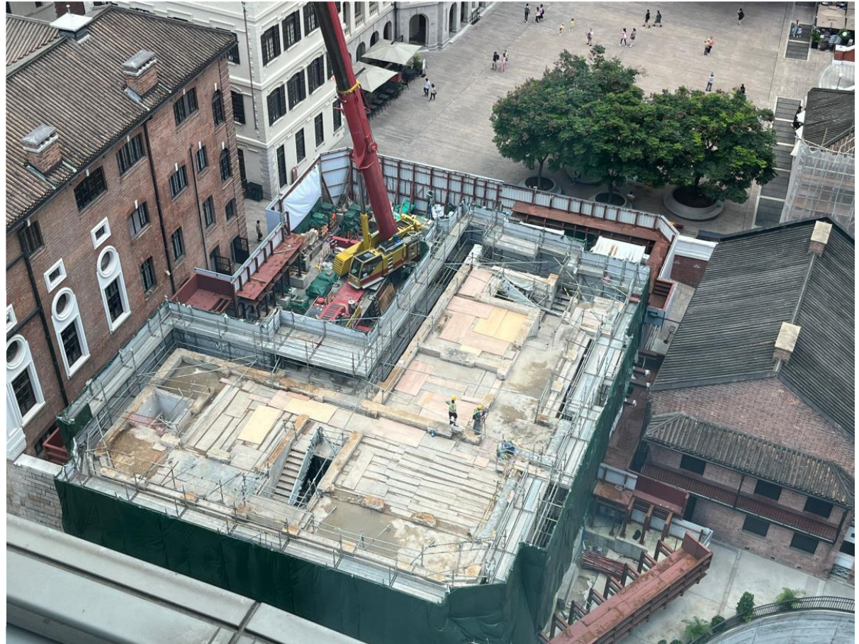
Figure 4 – Stage-completion of removal of unsafe building fabric (completion by June 2024)
