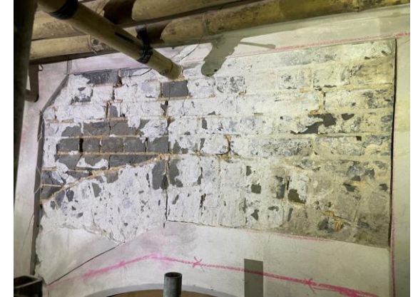
Location W1-2: View of brickwork condition after open-up
