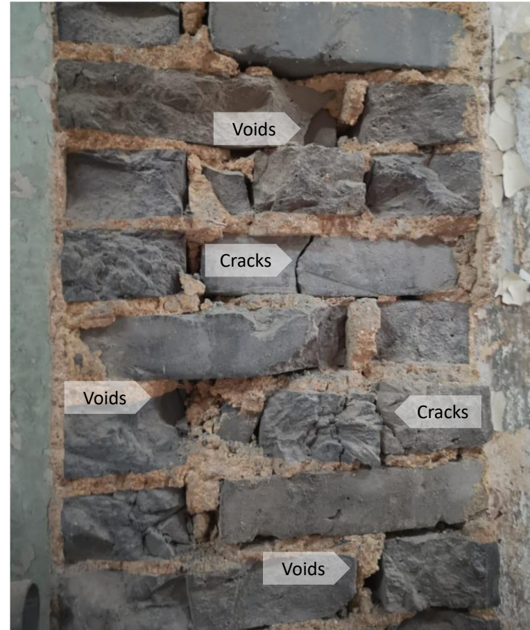
Figure 9 – Brickwork at door opening (section) showing substantial cracked bricks, voids and poor bonding in wall core (Location: Wall Zone W5 on 1/F)
