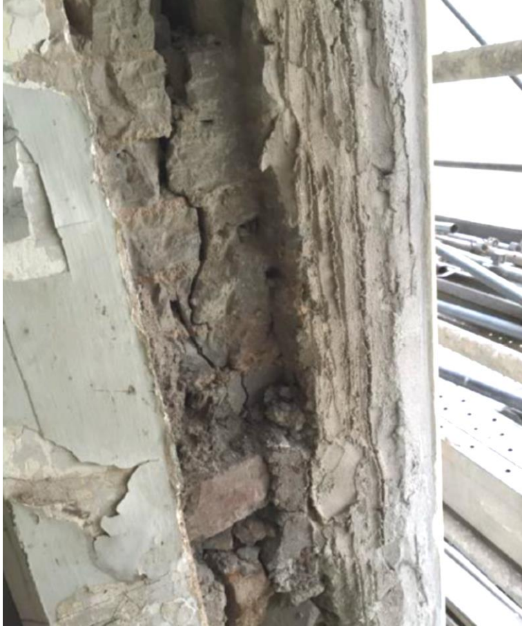
Figure 13 – (a) Cracks in brick pier noted after removal of window frame (Location: Wall Zone W4 on 1/F) (b) Failed pier stabilised by clamped timber boards (Location: Wall Zone W4 on 1/F)
