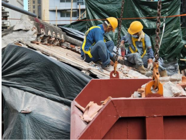
Removal of clay tiled roof coverings
