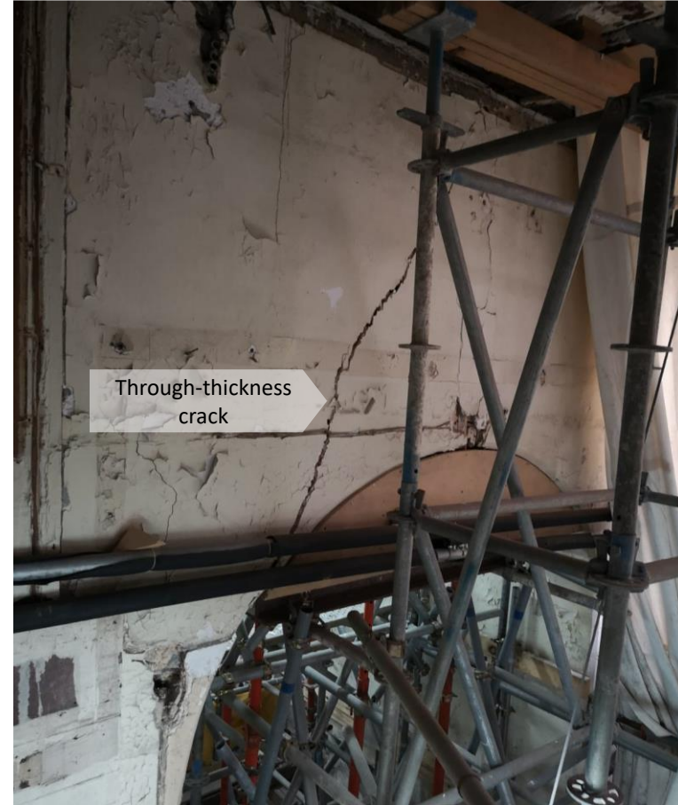
Figure 10 – (a) Poor bonding of brickwork, erratic in pattern and level (Location: Wall Zone W6 on G/F) (b) Through-thickness cracks in the west staircase portal (Location: Wall Zone W5 on 2/F)
