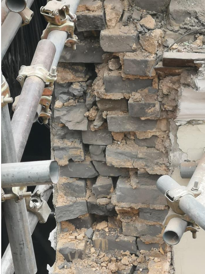
Figure 17 – Cracked bricks, voids and a lack of mortar at brick joints observed; individual bricks removed easily from main body of brick walls
