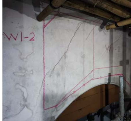
Location W1-2: View of render surface condition before open-up
