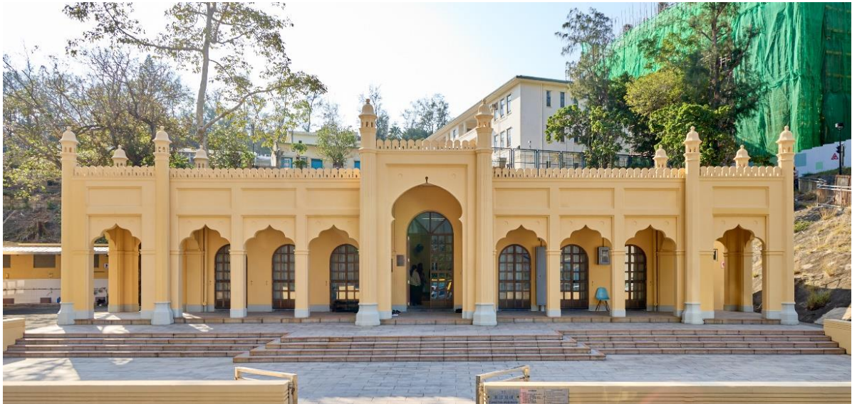
Front elevation of Stanley Mosque
