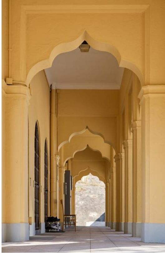
Open verandah with decorative ogee arches and moulding
