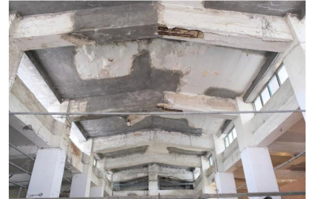
Fig. 132. Reinforced concrete roof slabs and beams viewing from the interior in 2020. 287
