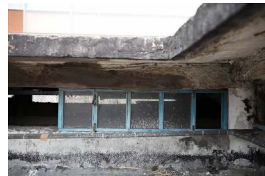
Fig. 90. Clearstory installed with timber framed window in 2020. 233
