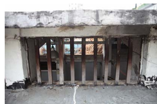
Fig. 91. Clearstory installed with timber grilles in 2020. 234
