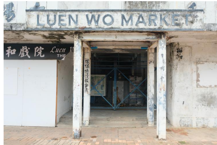
Fig. 101. Temporary steel structure under the entrance canopy in 2020. 246
