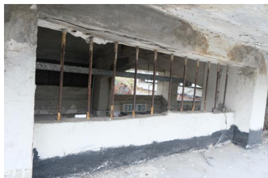
Fig. 89. Clearstory installed with metal grilles in 2020. 232
