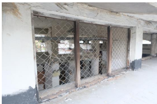
Fig. 87. Clearstory installed with wire mesh in 2020. 230
