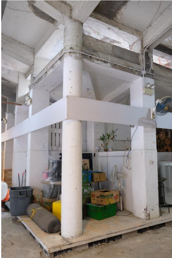
Fig. 134. Circular column (reinforced concrete) at corner and square columns (brick) in 2020. 289
