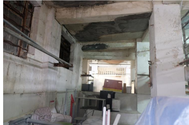
Fig. 100. Stall partition removed, with windows replaced by later metal windows at meat stalls in 2020. 245
