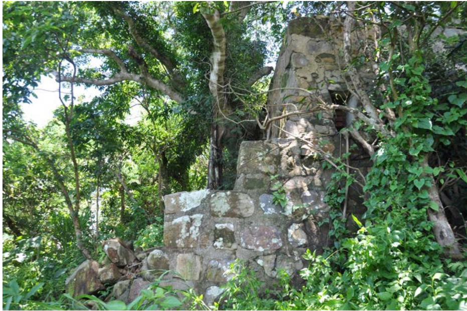
External view of protruding buttress at southeast corner of Paddock C18; also showing a possible draining hole at ground level (from inside), now sealed with red bricks, looking west.
