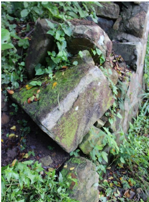
Heavily damaged buttress end
