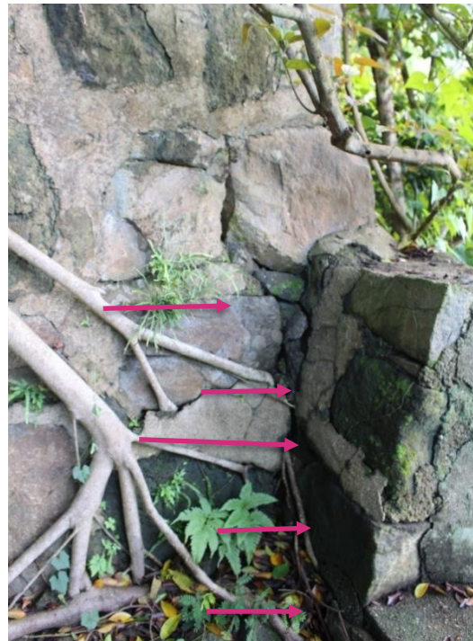
Buttress wall separating from main wall
