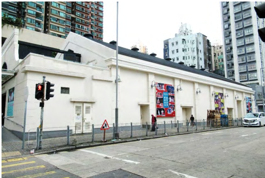
Fig. 54. Projecting cornice underneath the eaves and the pilasters at west and east elevation. (photograph by Author)
