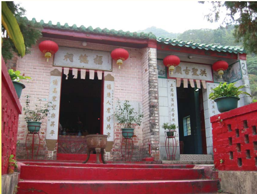
香港筲箕灣(近筲箕灣道8號)洪聖古廟及福德祠 Hung Shing Temple and Fuk Tak Temple, near No. 8 Shau Kei Wan Road, Shau Kei Wan, H.K.
