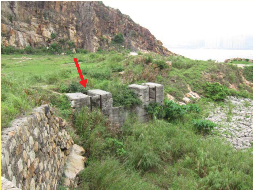
碎石機混凝土底座 Concrete Base for a stone crushing plant
