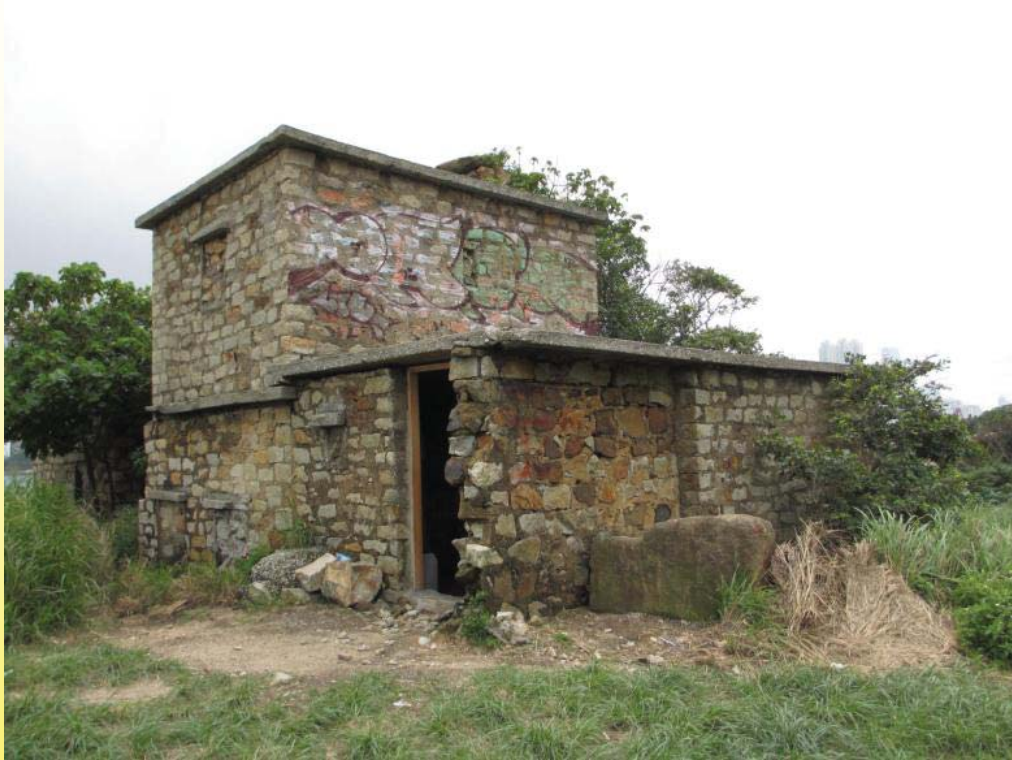
石屋（監工/守衛宿舍） Blockhouse (Overseer's Office / Watchmen's Quarters)
