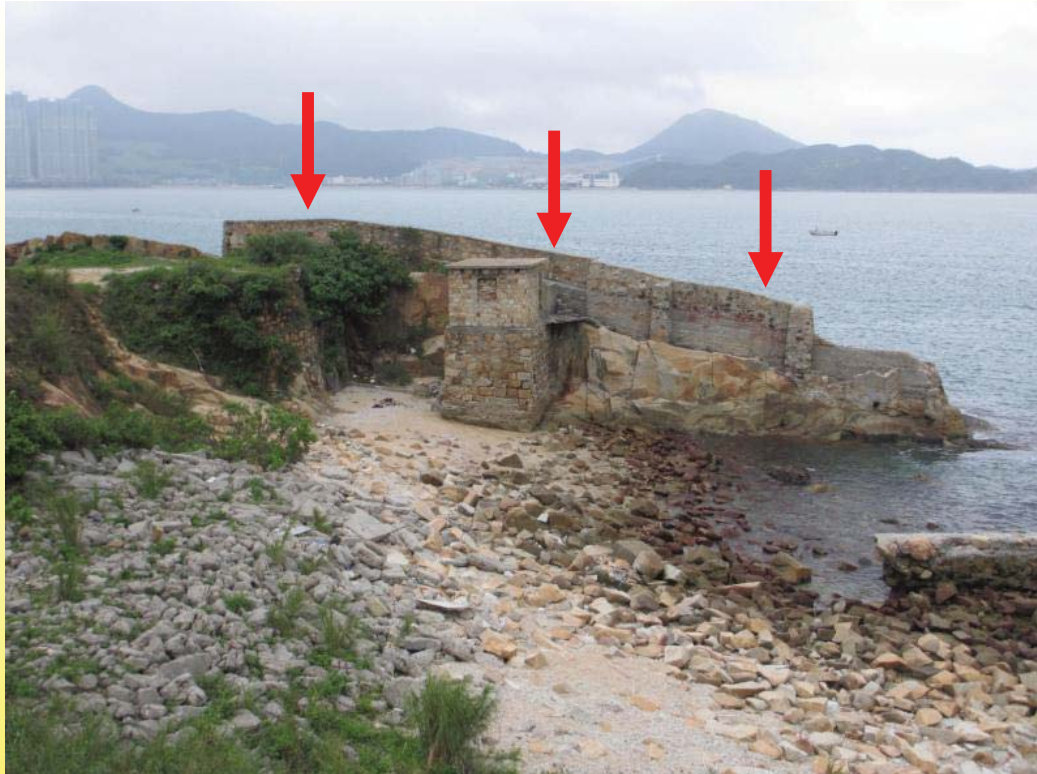
海堤（碎石堆存） Seawall (a site for stockpiling of crushed stone)
