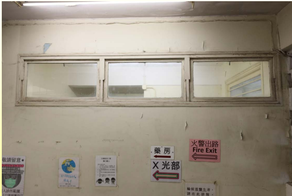
水平中心樞軸的楣窗及放置滅火筒的凹槽 Horizontal pivot fanlight windows and recess on the internal wall for fire extinguishers
