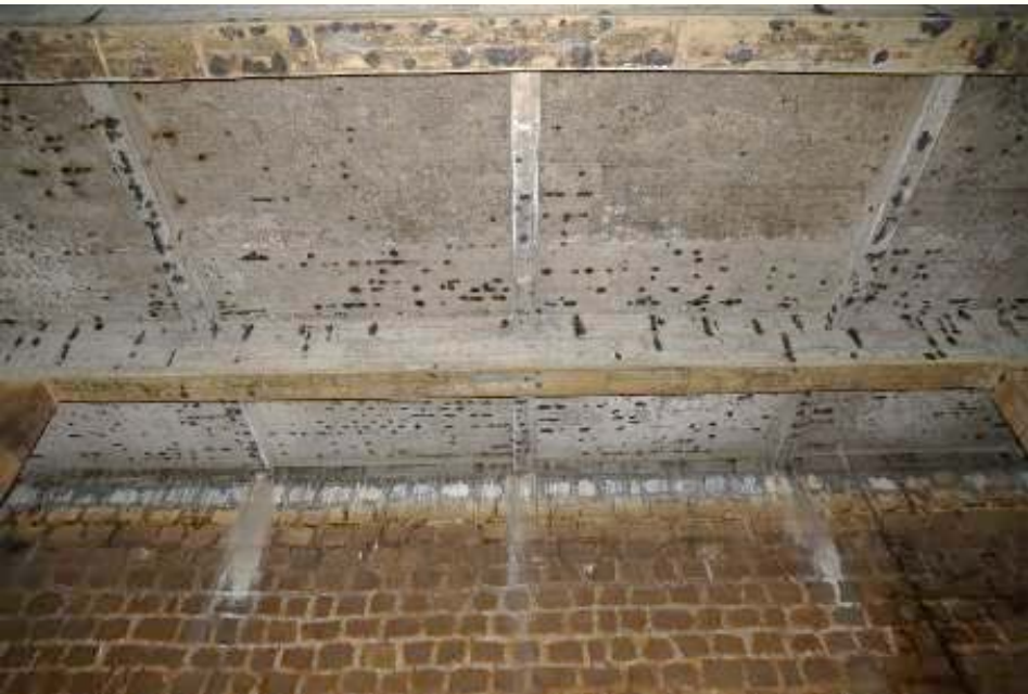
鋼筋混凝土樑板 (Reinforced Concrete Roof Slabs)
