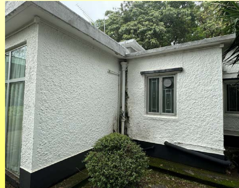
灰泥外牆 Stucco Walls
