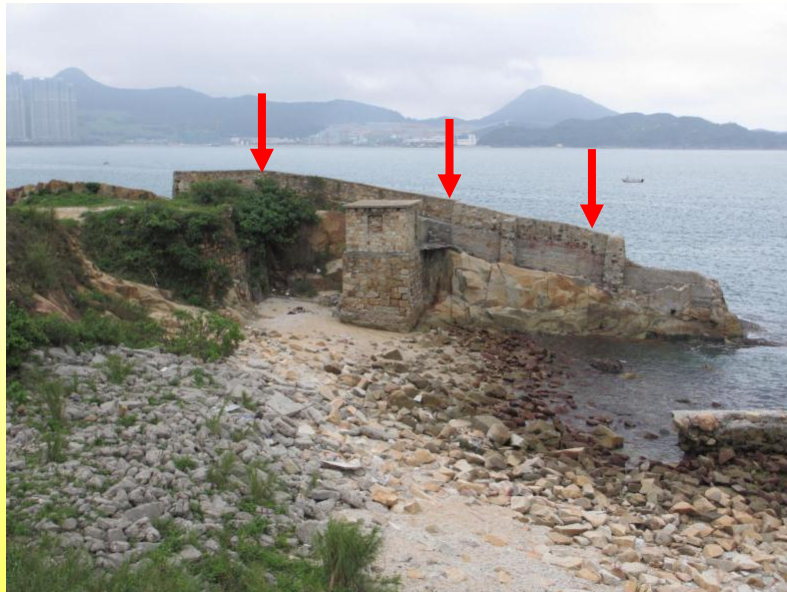
(7) Seawall (a site for stockpiling of crushed stone)
