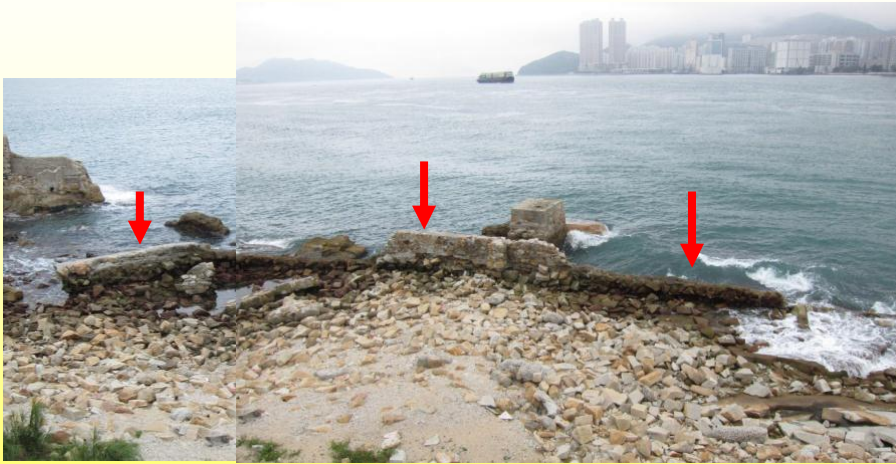
(4) Quay and Retention Wall along the southern boundary of the site
