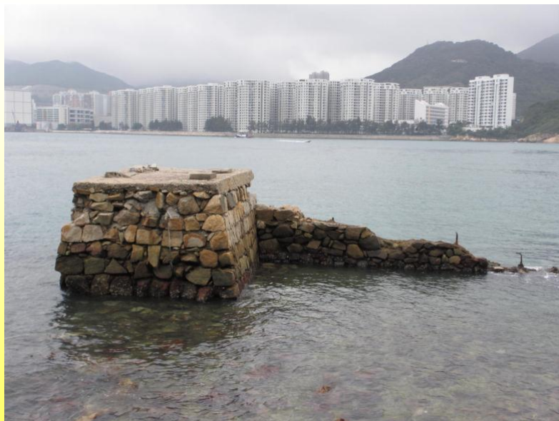
(3) Quay and Retention Wall at the western end of the site
