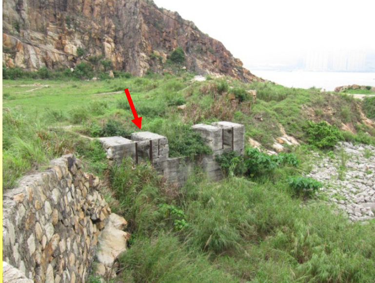
(12) Concrete Base for a stone crushing plant
